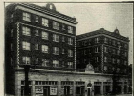
80,000 sq. ft. of STEELTEX FOR FLOORS strengthen and protect this attractive apartment building, 4011 Delmar Blvd., St. Louis, Mo. STEELTEX acts as a combined reinforcing and concrete form—saving time, labor, material, and money.
