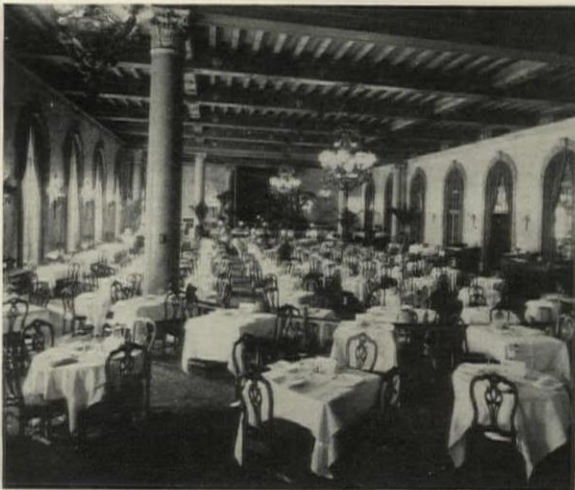
Dining Room Having Chandeliers and Brackets of the Candle Type. Local Table Lights are Provided
