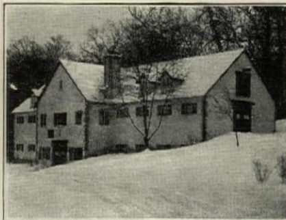
This is the most modern of stables—polo stables at the Dayton Country Club, Dayton, Ohio, architect, H. Lorenz. The backing of STEELTEX FOR FLOORS is of sufficient strength to afford safe walking surface, once the fabric has been attached to the joists.
