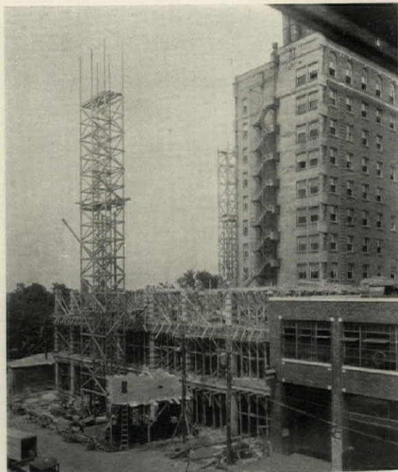
Building Designed and Constructed for Future Addition. Robert E. Lee Hotel, Winston-Salem, N. C.
