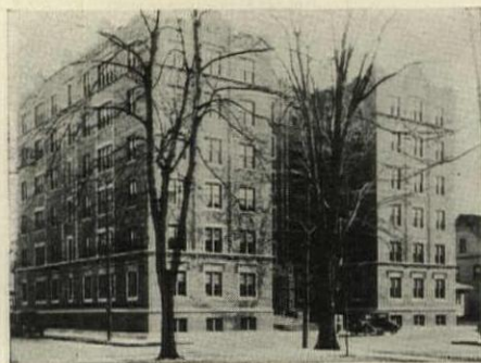
Park Lane Apartments, Hackensack, N. J., are guarded by Exide Emergency Lighting Batteries. Arthur E. Dore, Hackensack, N. J., Architect.
