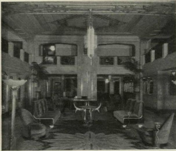
Modern Lighting Fixtures of Frosted Glass Panels. Central Fixture Equipped with 13 25-Watt Lamps.
