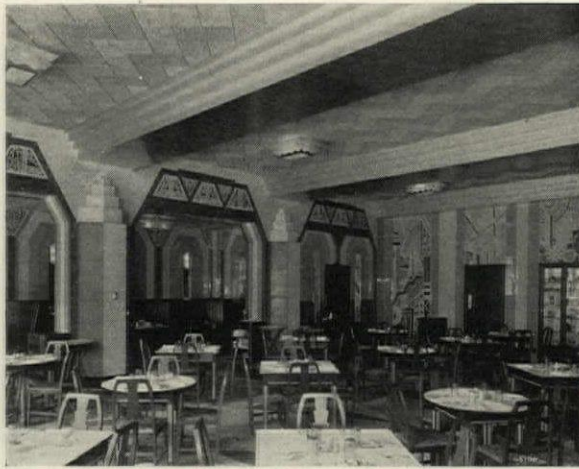
Sound Absorbent Fiber Board Ceiling in the Shorecrest Hotel, Milwaukee
