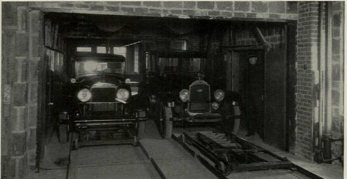
An Elevator Garage System which Permits Cars to be Locked by the Owners. Subsequent Handling and Parking are Accomplished by Means of the Trucks Shown
