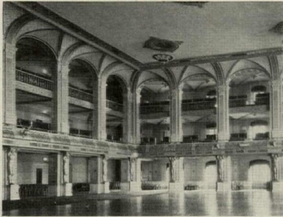
Ceiling of Acoustical Plaster in a Large Ball Room
