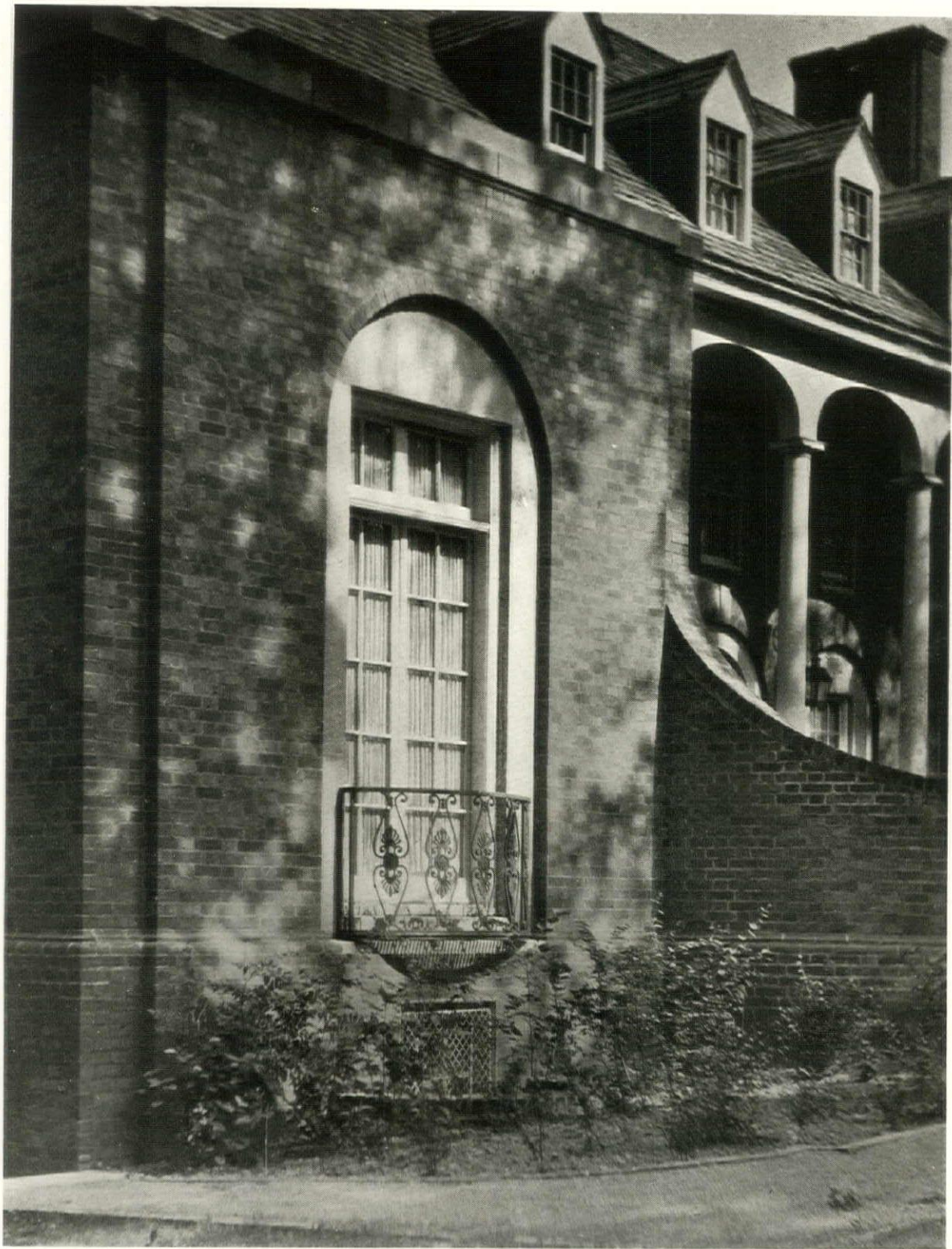
A WINDOW IN THE LEFT HAND WING WOMEN'S PHYSICAL EDUCATION BUILDING WEST VIRGINIA UNIVERSITY, MORGANTOWN DAVIS, DUNLAP & BARNEY, ARCHITECTS
