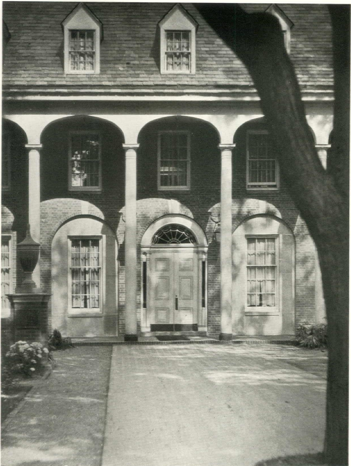
MAIN ENTRANCE DOOR AND PORCH WOMEN'S PHYSICAL EDUCATION BUILDING WEST VIRGINIA UNIVERSITY, MORGANTOWN DAVIS, DUNLAP & BARNEY, ARCHITECTS
