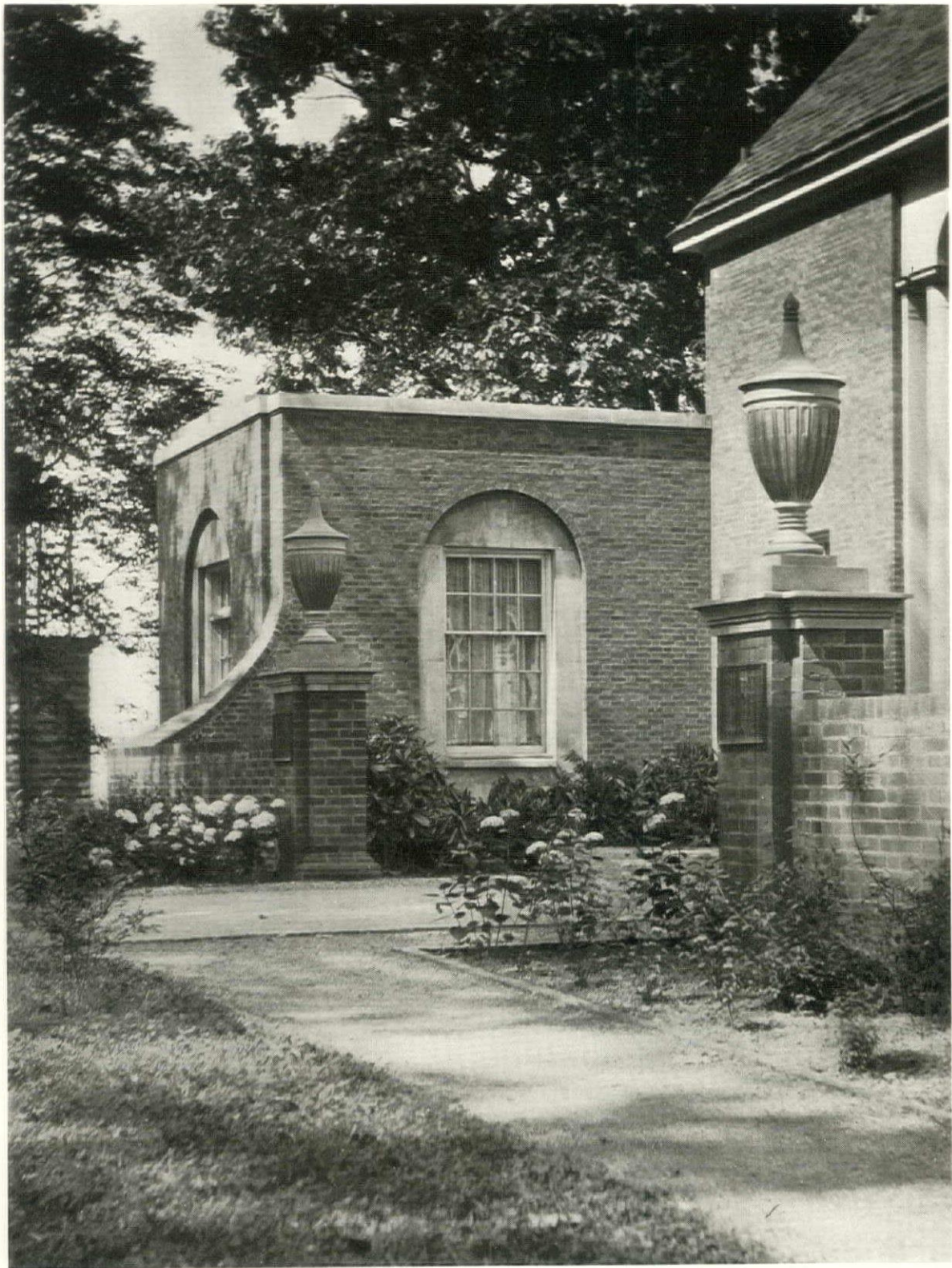
DETAIL OF THE ENTRANCE COURT WOMEN'S PHYSICAL EDUCATION BUILDING WEST VIRGINIA UNIVERSITY, MORGANTOWN DAVIS, DUNLAP & BARNEY, ARCHITECTS
