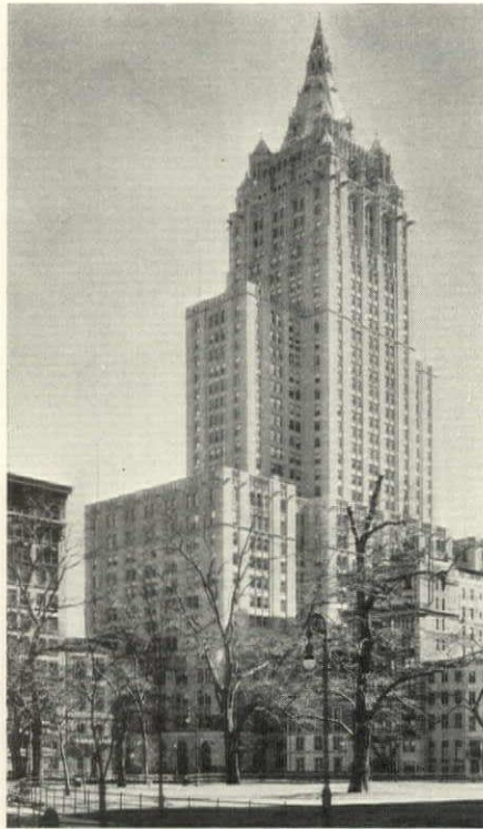
New York Life Insurance Building, New York. Cass Gilbert, Architect
