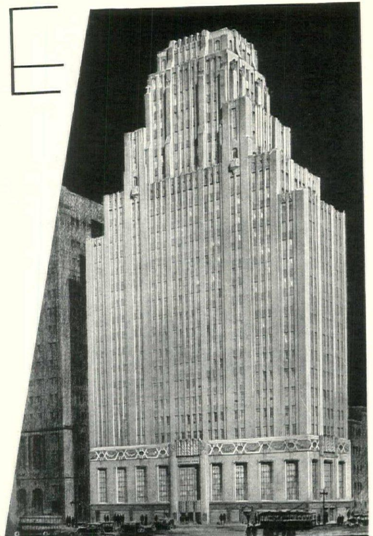
MARKET STREET NATIONAL BANK BUILDING, PHILADELPHIA RITTER & SHAY, Architects and Engineers WM. STEELE & SONS CO., General Contractors AMERICAN BRIDGE CO., Fabricators
