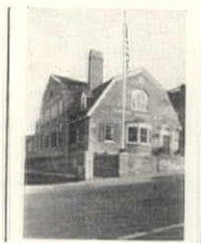
Clinton, Mass., Savings Bank; Hutchins & French, Archts., J. E. Chatman, Engr., Lynch & Woodward, Heating Contrs.
