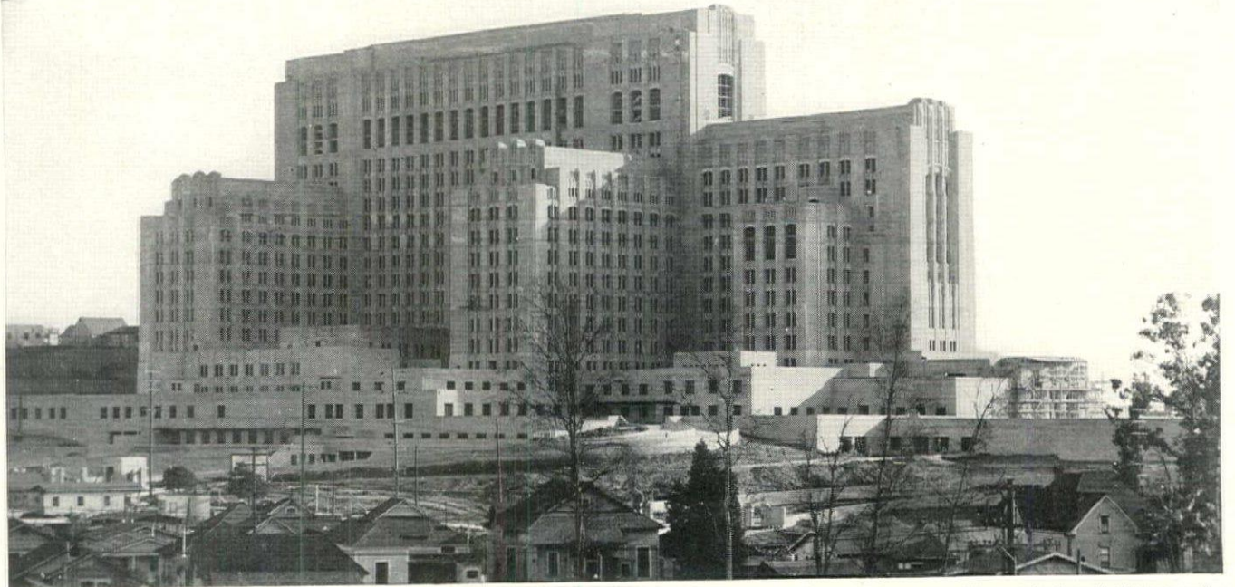
Los Angeles County Hospital, Los Angeles, California; Architect—Allied Architects of Los Angeles; General Contractor—Weymouth Crowl; Waterproofing Contractor—Owen Roofing Company.
