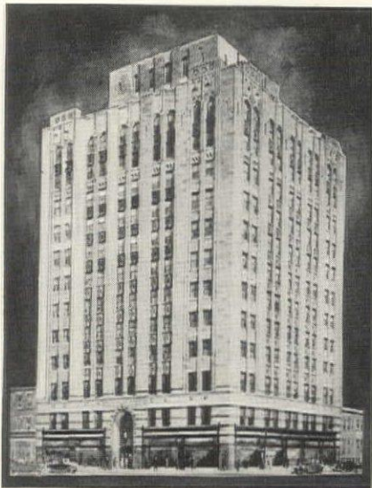
Roofed with ATP AMERICAN BANKERS INSURANCE CO. BUILDING Cass and Ohio Streets Chicago, Illinois Architects: Childs and Smith General Contractor: E. P. Strandberg Co., Inc. Roofing Conrt: Chicago Waterproofing & Roofing Co.
