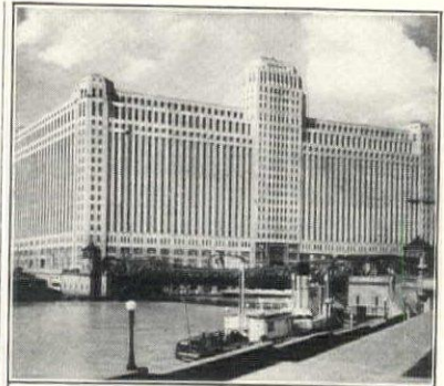
Merchandise Mart, Chicago. Graham, Anderson, Probst & White, Architects. U. S. Gypsum Co., Sound Insulating Contractors.
