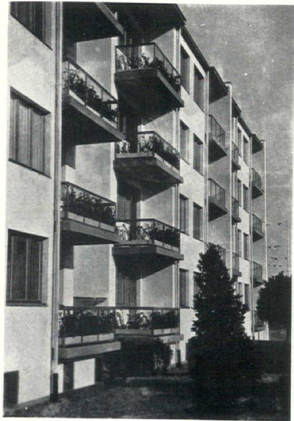
Group 6. West Elevation Walter Gropius, Architect
