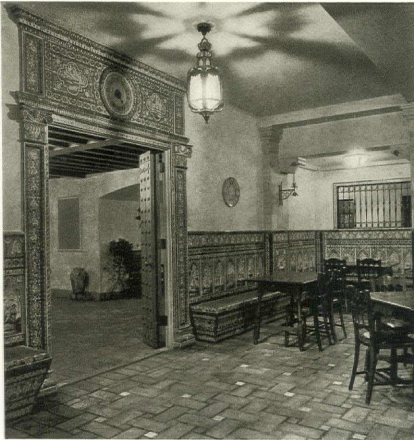
DOORWAY BETWEEN CAFETERIA AND BASEMENT LOBBY. BELOW, VIEW OF CAFETERIA
