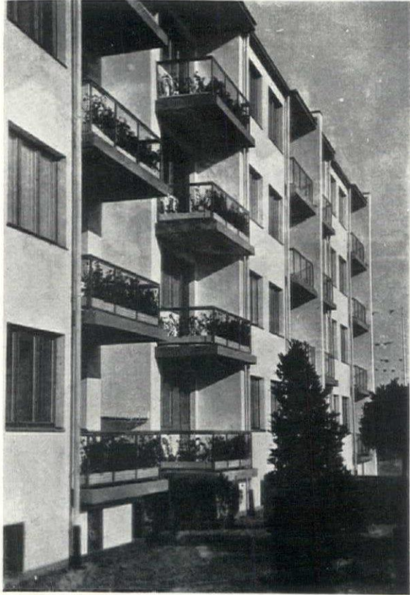
Group 6. West Elevation Walter Gropius, Architect
