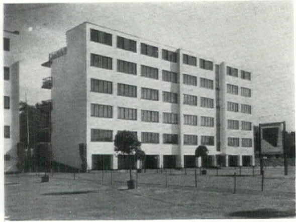
Group 5. West (Rear) Elevation Walter Gropius, Architect
