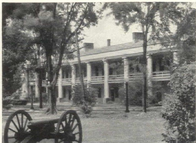
Still serviceable for years to come, the Tidewater Red Cypress on Old Baton Rouge College has already weathered many a decade of sun and rain. Photograph by Tobbs & Knoll
