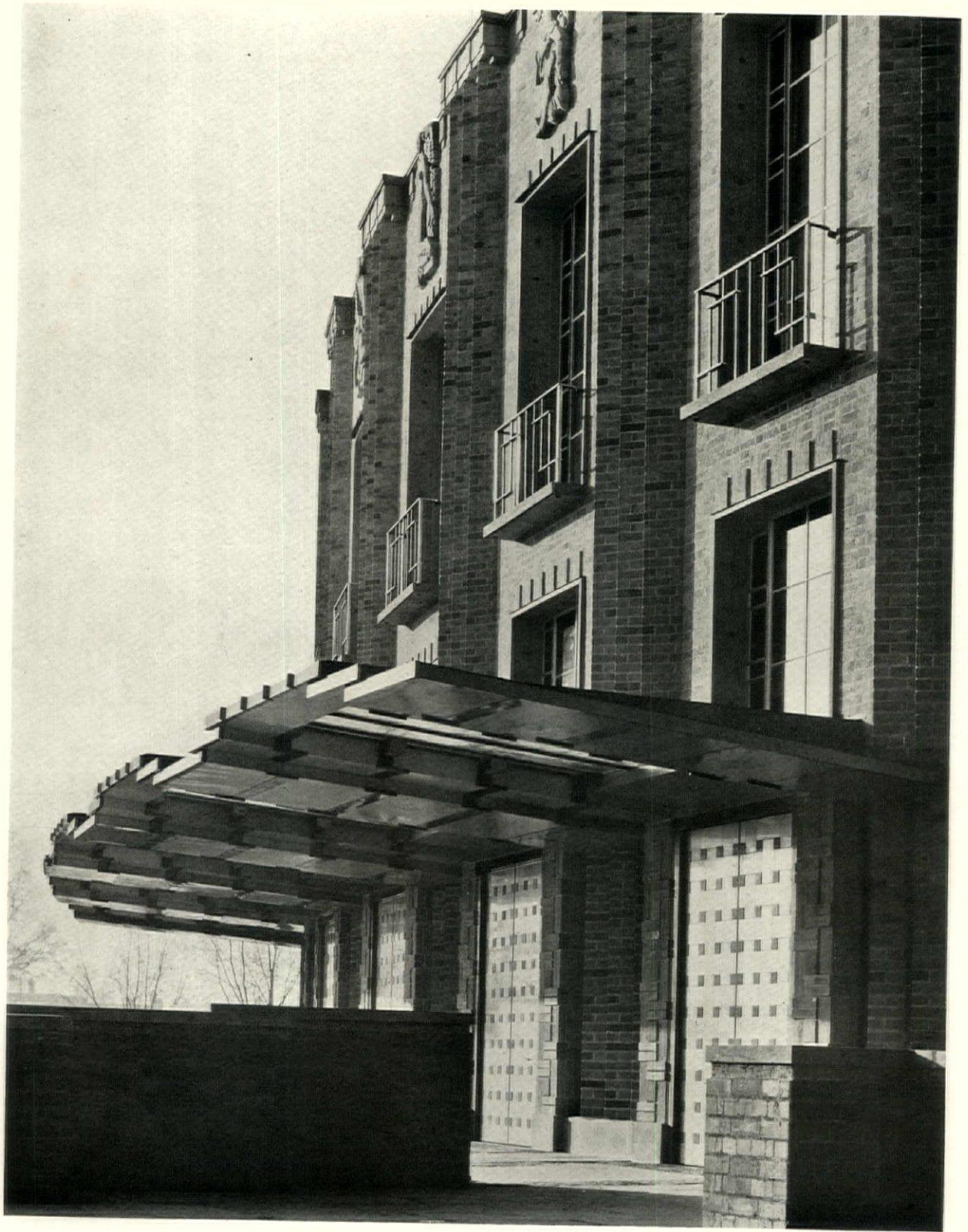
NORTH ENTRANCE AND MARQUEE
