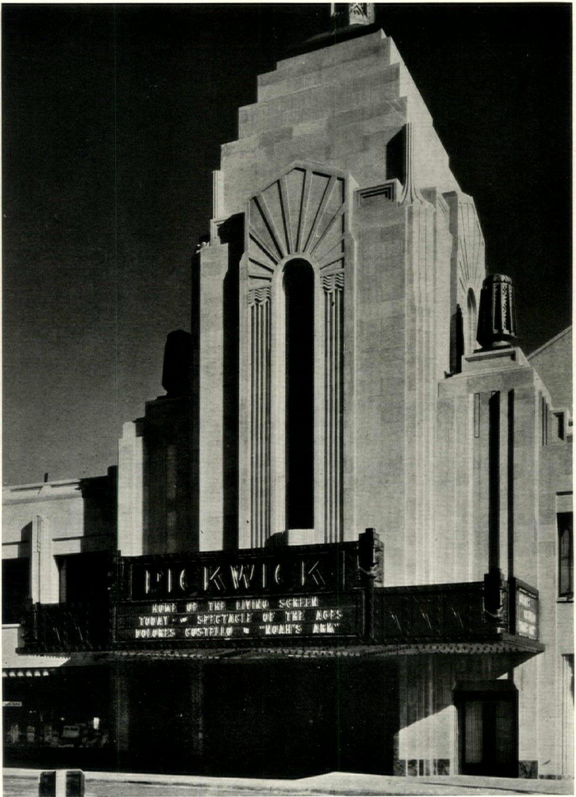
PICKWICK THEATER PARK RIDGE, ILLINOIS R. HAROLD ZOOK, ARCHITECT
