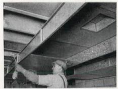
Even the trunks are standardized in the fully pre-fabricated Tempered-Aire duct system
