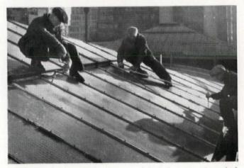
Workmen recently replacing worn-out skylight frames on the roof of the Pennsylvania Station, in New York, with Monel Metal. See what weathering did to the old frames in the foreground.
