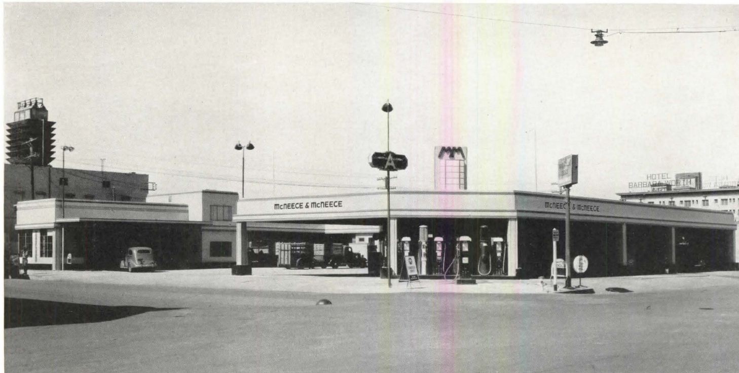
SERVICE STATION FOR McNEECE & McNEECE, EL CENTRO, CALIF. DESIGNED BY NIGG ENGINEERING CO.
