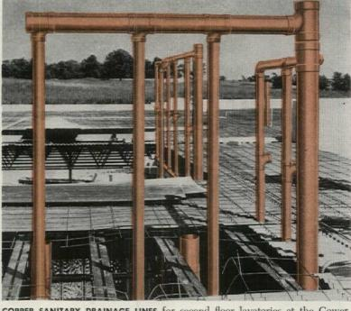
**COPPER SANITARY DRAINAGE LINES** for second floor lavatories at the Gower School. Light weight of copper tube and ease of making solder joints save many dollars on multiple installations like this. Compact assemblies eliminate wide plumbing walls, give greater usable floor area.
