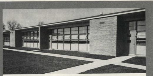
NEWER SCHOOLS GO VISION-VENT . . . Truscon's fast, economical window-wall construction. It is com pletely flexible. You can select practically any type of window—double-hung, architectural projected, intermediate projected. Arrangement of fixed lights, operating lights, insulated panels is completely interchangeable. In either steel or aluminum. In designing low-cost schools, investigate Vision-Vent St. Jude's School. Architect: Johnson & Bouton; Contractor: Victor R. Beauchamp Associates, Inc.
