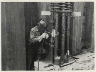
NO. 185 HIGH STRENGTH REINFORCING BARS used in column verticals are electrically butt-welded in basement story adjacent to steel sheeting. To accomplish the weld, the lower bar is furnished with a square cut end and the top bar is beveled at 45 degrees from each side to form a chisel end. Clamps are used to hold bars in alignment.
