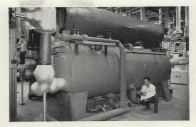
**MAINTENANCE COSTS TO DATE— ZERO!** The Allen Company uses two York machines—a 230-ton unit serving 45,000 sq. ft. of office and cafeteria space, a 170-ton unit for process water cooling. Three small pumps and motors are the only moving parts in the entire system.
