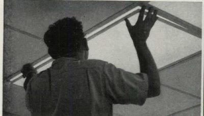
The discomfort of direct and reflected glare is reduced with Fiberglas Polarizing Light Panels, which also conform to the established ceiling module. The Fiberglas Polarizing Light Panel combines the two most sought-after properties in lighting control—cutting off direct glare like a lens or louver . . . and reducing reflected glare like a diffuser. The textured appearance of Fiberglas Polarizing Light Panels provides interesting, decorative effects which are architecturally neutral.
