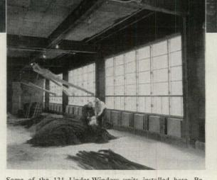
Some of the 131 Under-Window units installed here. Because of the highly efficient way in which it blankets the cold outer walls with warm air, this attenuator is ideal for the climate, where cold wind, ice, and snow vigorously bear in upon the buildings much of the time.
