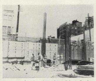
This photo shows first and second story column verticals extending above the basement floor after having been butt-welded to the dowels in caisson tops. Bars are No. 185 high strength types furnished by Republic Steel.
