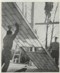
Four-man team from Boss Glass Company, Caldwell, N. J. enclosed 1000 sq. ft. of wall area a day. Men had never installed Kalwall before. 14' x 4' panel unit is so light one man can push it upright. Panels are held in place by channels bolted to floor and roof.
