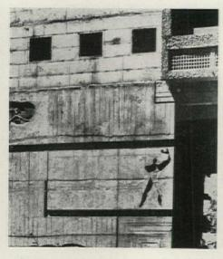
The church's concrete (right) was rather too well finished, thus shows every little crack and stain-including herringbone cracks around glass slots caused, possibly, by different coefficients of expansion in the concrete and glass. Le Corbusier's béton brut, as at his apartment building in Nantes (above), is deliberately rough from the start and looks weathered right away.
