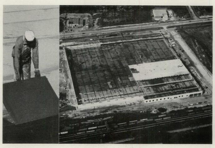
Photo shows part of 450,000 square-foot, Gold Bond Poured Gypsum Roof Deck in place on F. N. Burt Co. factory, Cheektowaga, N.Y. Deck was insulated with Gold Bond Roof Board.
