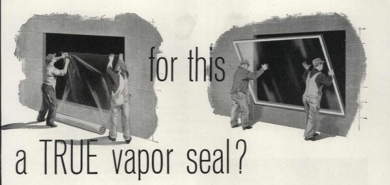
It is fortunate that within the last decade the building industry has recognized the need to install a vapor barrier between the site and structure . . . unfortunately, the building industry has been guilty of the promiscuous use of permeable materials under the guise of vapor barriers. It is a known fact that asphalt saturated felts and building papers, duplex papers and plastic films are all highly permeable and should not be considered as effective vapor barriers.
