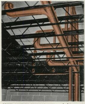
**COPPER SANITARY DRAINAGE LINES** roughed-in among structural members at Gower School. This space-saving installation would have been impracticable with heavy, bulky pipe requiring threaded or caulked joints.
