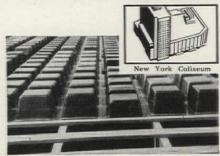
Specifiers of reinforced concrete construction find GRID SYSTEM highly effective and versatile, for heavy-duty floors and ceilings. Economical GRID SYSTEM construction permits maximum column-free spans, by removing dead-load concrete. Use of removable interchangeable GRID domes offers great flexibility in layout of utilities. GRID SYSTEM construction carries maximum loads, approaches 100% concrete efficiency in thousands of buildings across the country.\*
