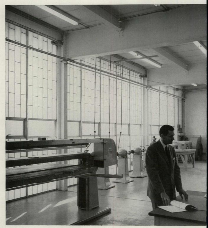
Only 113 Kalwall panels were needed to enclose the entire 6000 sq. ft. Edburgh plant. Architect Ian M. Horne, who designed the building, reports, "the interior is filled with so much glareless light, daytime use of electric lights will seldom be needed." Installed cost of translucent Kalwall was considerably less than bids submitted for other curtain wall systems,
