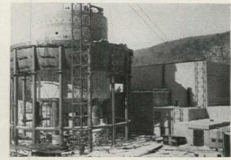
In New England, Yankee Atomic Electric Co. is building this 134,000-kilowatt atomic power plant (above) at a cost of about \$50 million. The reactor, designed by Westinghouse, is housed in a ball on stilts (see photo, right), so that railroad cars can move beneath it to carry off waste materials.
