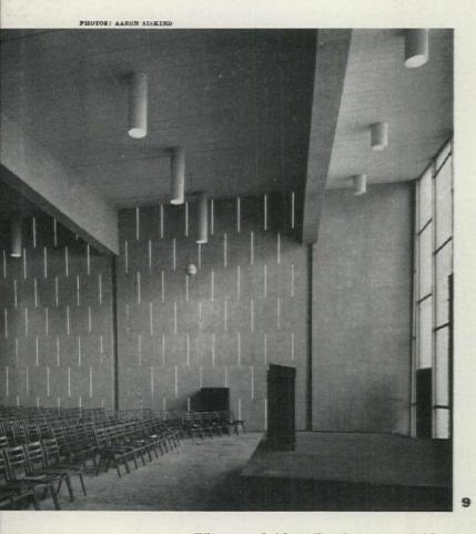
Tilt-up sandwich walls of concrete (with a glass-fiber core) are penetrated by regularly spaced slots, filled with cast glass. The lighting effect on the inside is highly successful during the day and just as successful from the outside at night, when the slots of light shimmer in the darkness. Danish chairs are a pleasant touch in this austere room.
