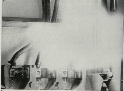
Dangerous arcing with open knifeblade switches
