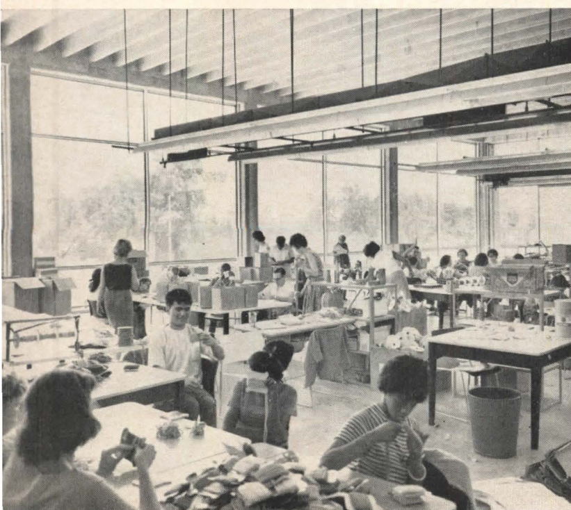
Student therapy building (3, and top left) has cafeteria, auditorium, swimming pool, therapy rooms. Upper floor (middle) looks out toward administration (2) and classroom units (1). Construction throughout is designed for low cost and low maintenance. Workshop (5, and below) is a concrete frame building, with parking at ground level and a precast roof of 60-ft. clear span. Construction costs for the workshop building were well under $10 per sq. ft., says Barnstone, probably between $7 and $8 per sq. ft. Total costs averaged $16.50 per sq. ft.
