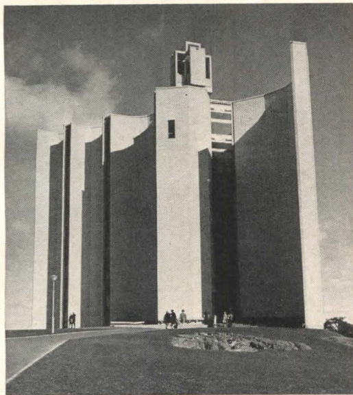
The brick-faced concrete "chutes" that enclose the Tampere church rise on a low hill at the end of the town's main street (above). Inside (left), their bare concrete surfaces show subtle gradations in brightness as they splay outward from full-height windows.
