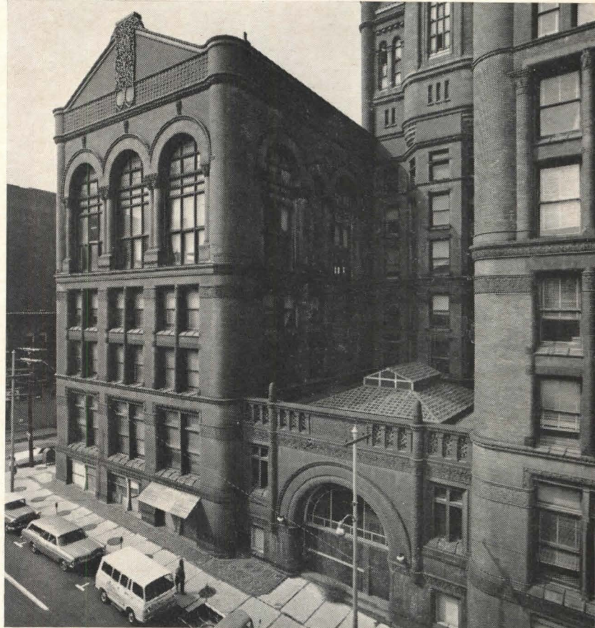
At the top of the west wing (facing page), arched windows and a gable decorated with terra cotta indicated the location of the grain trading hall (bottom right). The tall windows and coffered ceiling of the hall had been obscured with peeling black paint. The main entrance to the building, between the two wings (below right), was a low-springing brick arch, surmounted by a balustrade with terra cotta ornament (left).
