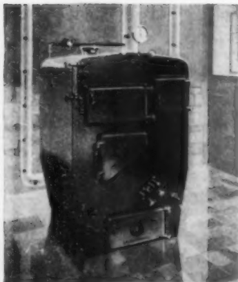
Shown above is the newest style of Spencer cast-iron sectional heater, for any home and for small business buildings, furnished with or without enameled steel jacket.
