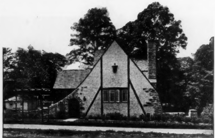
An interesting feature of some of our modern houses is the free use that is made of architectural precedents. In this case false half timber construction has been used to decorate a cottage
