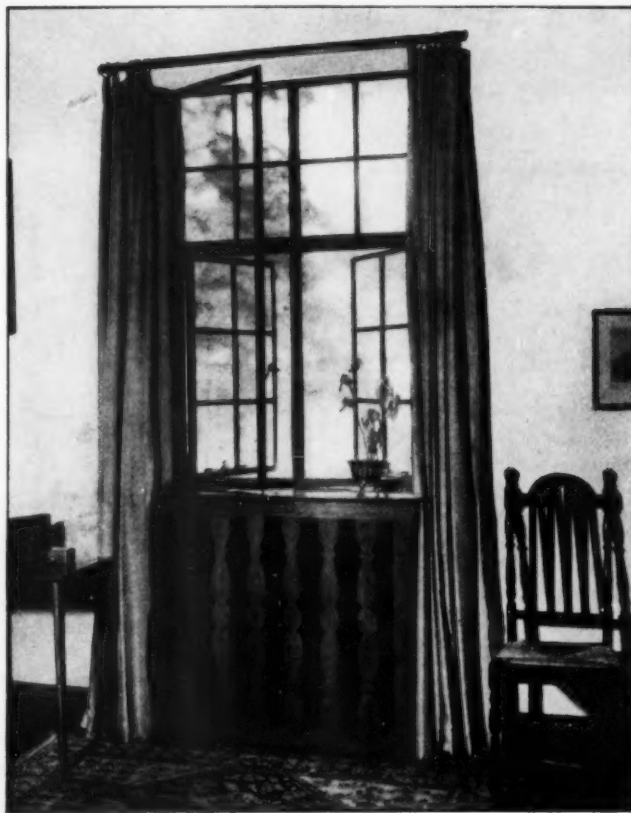
The carved wood grille adds a distinctive decorative touch to the entire room, at the same time effectively concealing the radiator
