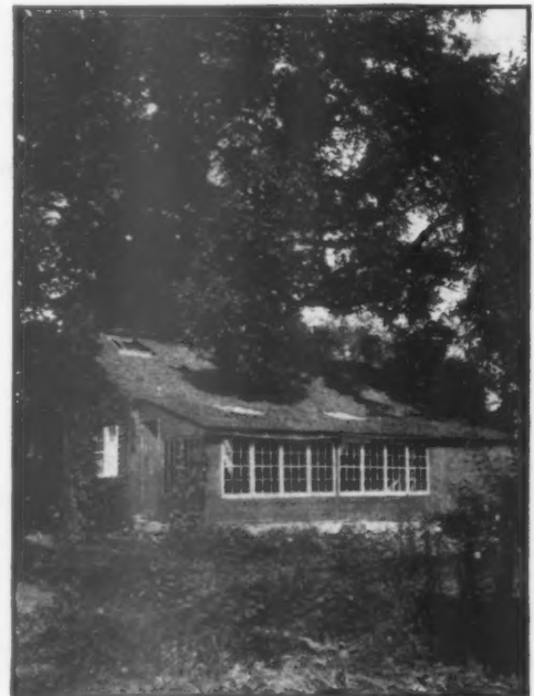
Here will be seen the addition that was made, which does not disturb the old roof line
