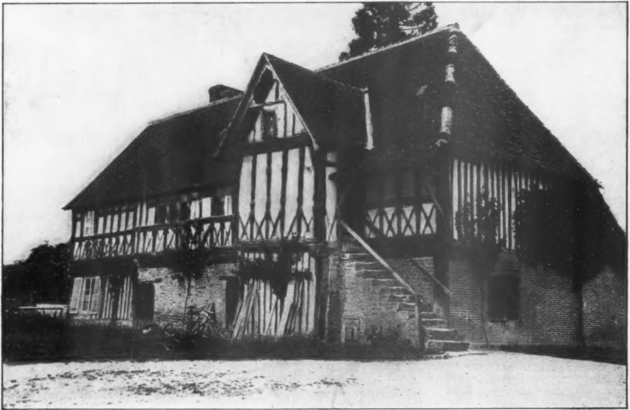
One difference between the French and English style of half-timbering seems to be that the French tried to use theirs decoratively at the same time that they employed it for structural purposes. The English on the other hand rarely, particularly in the early work, sought to make a pattern of the half-timbering. Our modern tendency is to use half-timbering decoratively, but not structurally
