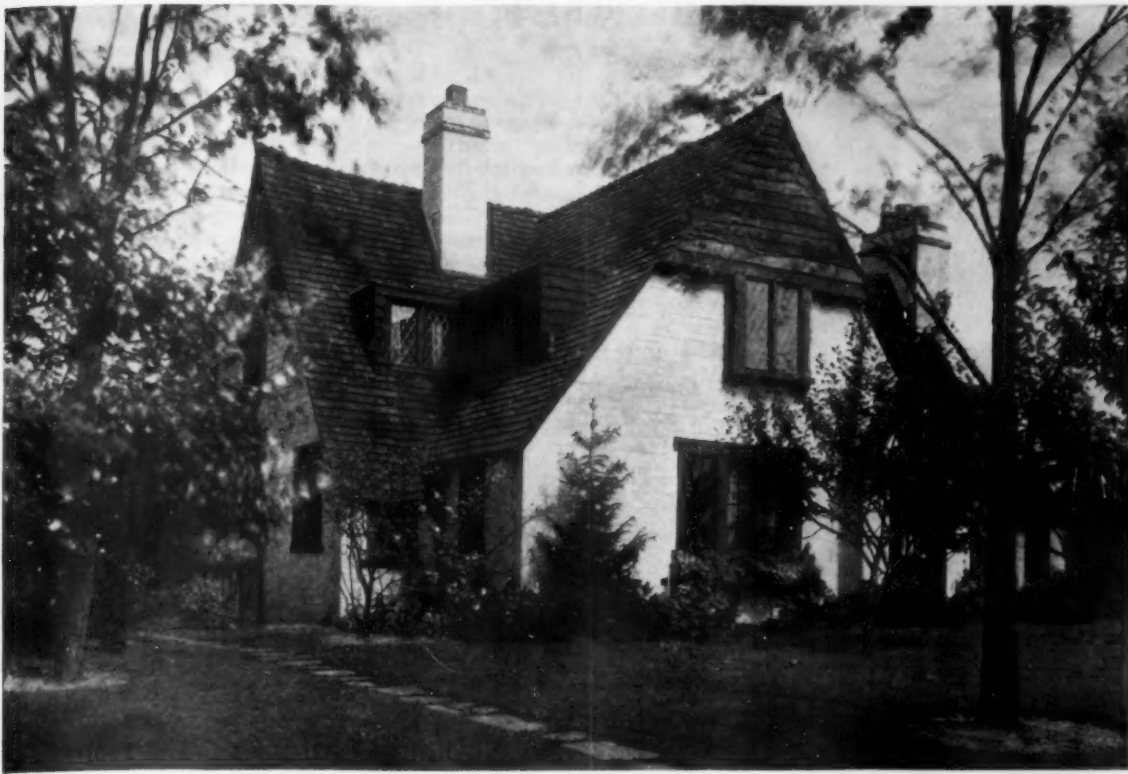
Concrete masonry residence of Clarence E. Day, Architect, Detroit, at Lake Angelus, Michigan. The walls are of variable sized units, producing a surface that is both interesting and effective.
