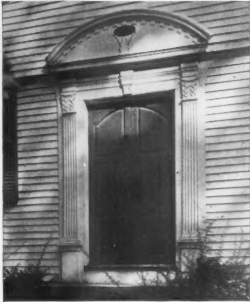
Doorway of a house at Farmington, Conn. Built of White Pine in 1690, and standing today
