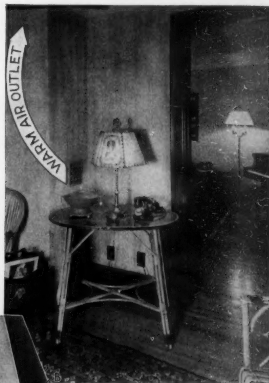
Heatilator Fireplace in the model steel frame house by Emil F. Kotz, Syracuse, N. Y. Cold fresh air enters the Heatilator from beneath the floor—an ideal ventilating arrangement. Part of the warm air leaves from the grilles shown above the mantel, and the rest through a grille in the sun porch, which makes the porch warm in winter. Grilles can easily be carried to the upper floor if desired. At left: The Heatilator as delivered, ready to install. "A" shows one of the cold air intakes; "B" shows one of the warm air outlets.
