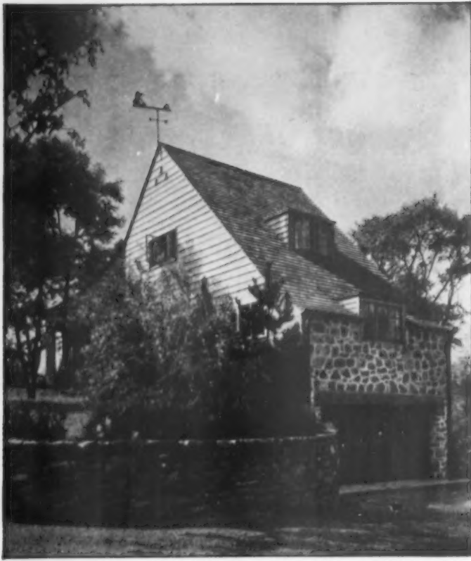
The land slopes from the front to the street level in the rear of the house, making it possible to place the garage in the basement
