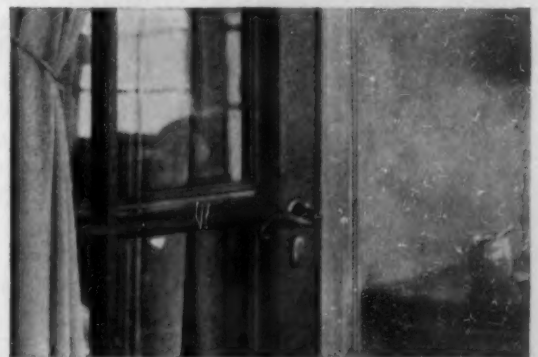
A Sargent lever handle in the Yarmouth design, used on interior as well as certain exterior doors, gives a graceful and unusual touch, thoroughly in agreement with the dwelling.
