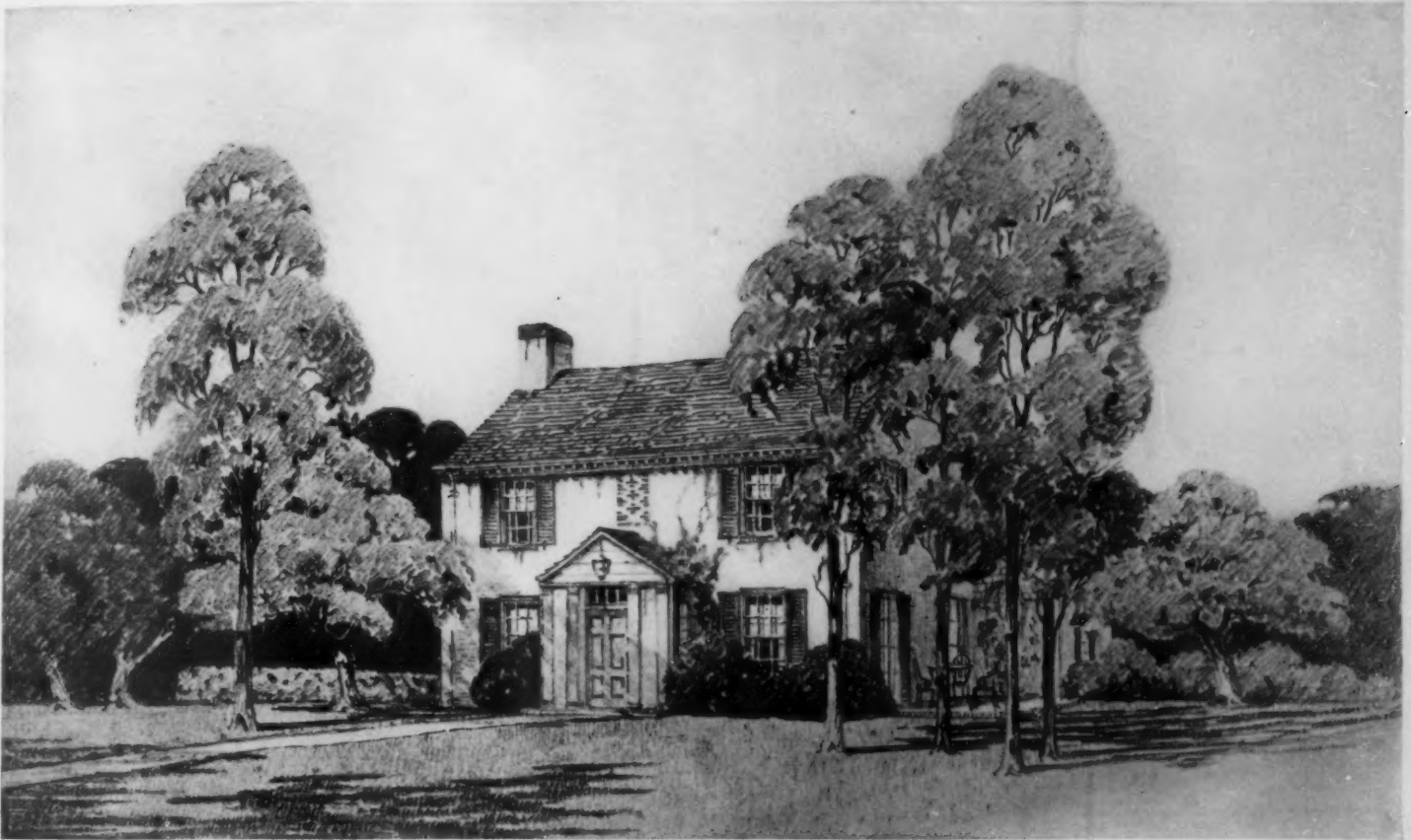
This simple house of brick contains 25,000 cubic feet and cost $11,250 to build. The style is a pleasant variation of the traditional Colonial or Georgian. The charming entrance feature, with its delicate pilasters and well-designed lantern, and the brickwork pattern on the wall above lend beauty to this façade. A French door in the living room opens on a flag-stoned terrace. The garage is set two steps below the level of the main house and is entered through a door in the back hall. There are three masters' bedrooms, one of which, the small one, might be used as a sewing room, a nursery, or an upstairs living room and converted into a guest room when necessary. The maid's room and bath is over the garage.
