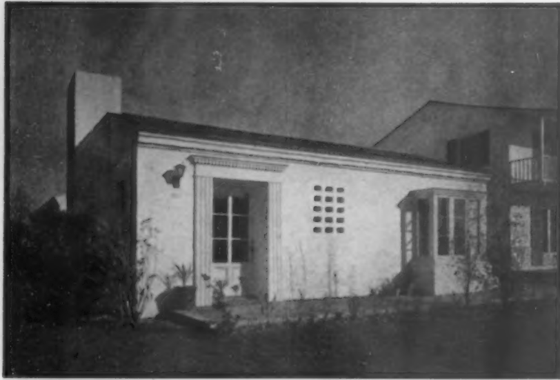
Above is shown the front elevation of the one-story house at 4125 Edgehill Drive, Los Angeles, designed by Gordon B. Kaufmann, architect. The floor plan is shown at the left. The door into the living room and the dining room bay show in the photograph. The two-story residence which appears at right is on an adjoining lot
