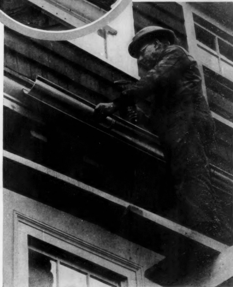
Installing Copper chimney flashing to prevent leaks. The use of materials less durable than Copper for service such as this is costly.
