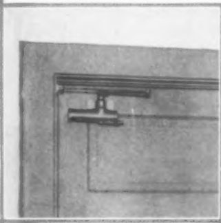
Spring door closers that control the speed of the closing door and prevent slamming are made in models for doors of varying weights. (P. & F. Corbin)
