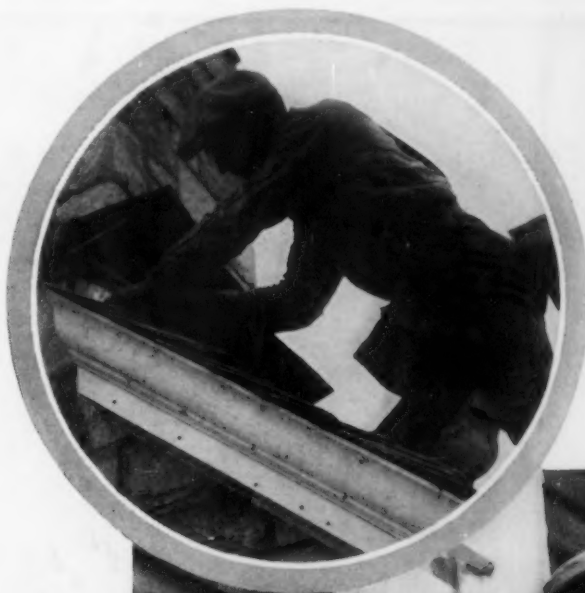
Installing Copper chimney flashing to prevent leaks. The use of materials less durable than Copper for service such as this is costly.
