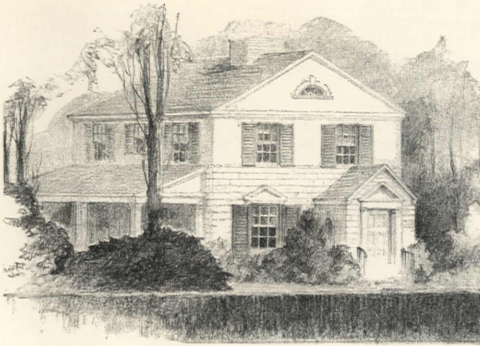
The house was stripped of all its toboggan slides and false side whiskers and its true beauty was brought out. Being a bit too box-like in shape it was made lower and the horizontal lines emphasized, giving it a lot more character
