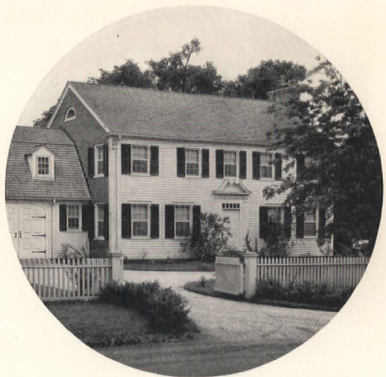
House at Naugatuck, Conn. Architect, Fred A. Webster, Waterbury Conn. Front and rear walls finished with Cabot's DOUBLE-WHITE Collopakes, blinds stained with Cabot's Creosote Shingle and Wood Stains.
