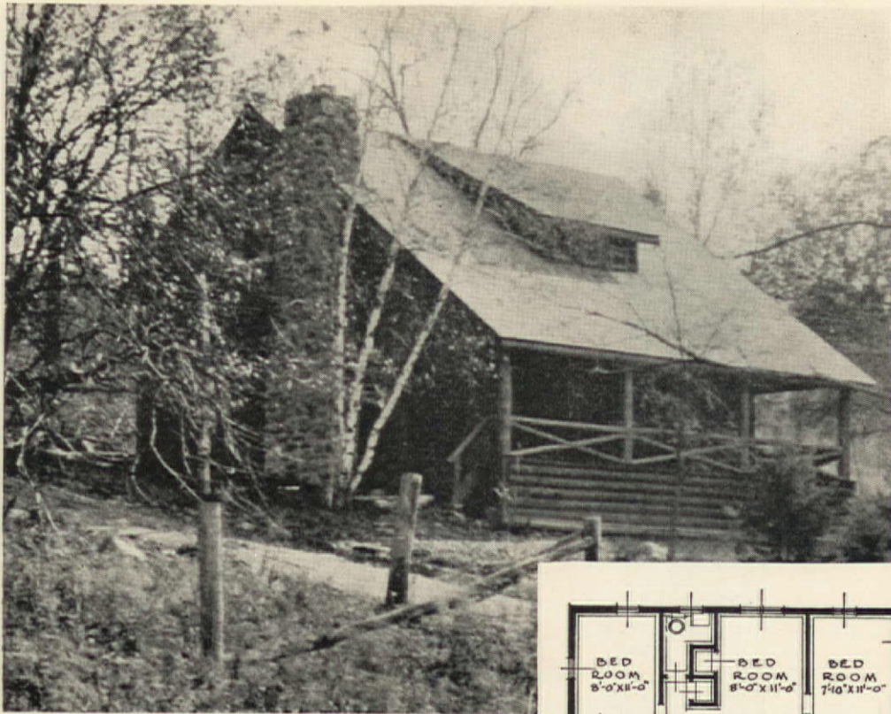
Log cabin of Mr. F. W. Scutt, Candlewood Lake Club, Connecticut. The chimney and fireplace, desirable features of the cabin, do not show on the floor plans but may easily be incorporated. The balcony off the living room provides additional sleeping quarters without actually giving the exterior effect of a second floor. Courtesy, Adirondack Log Cabin Co.
