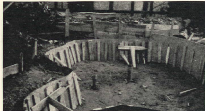
Linoleum braced with wood making the concrete form
