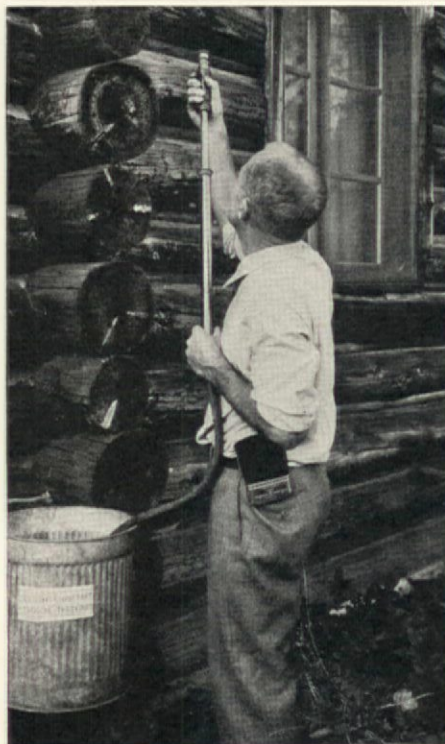
If the bark is removed from the logs they can be stained an attractive color by spraying with a mixture of one part of creosote to exactly three parts of kerosene
