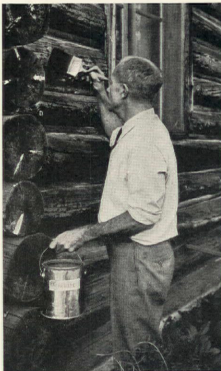
Painting or spraying the log cabin or rustic furniture where the bark is removed with crude pyridine will safeguard them against destruction of boring insects
