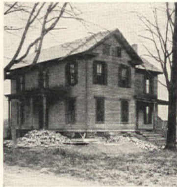
The house before remodeling
