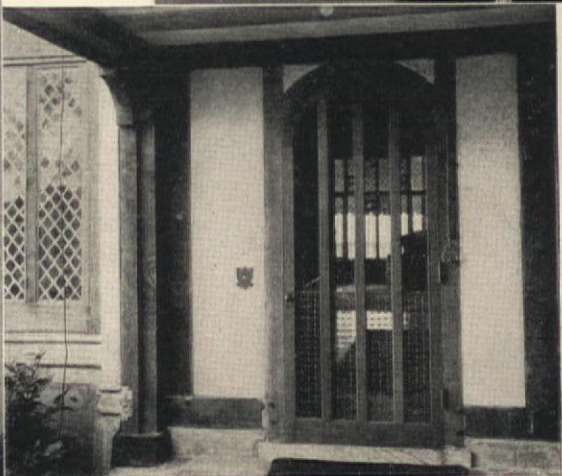
Blinds and screens may well conform to the architecture of the house as shown by the Higgin screen door above which was designed to conform to the original door
