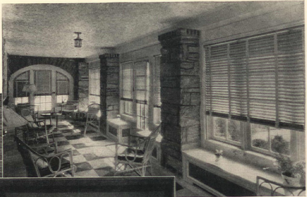
Below: The Fenestra "Fenwrought" casement is opened, closed, and securely locked without opening the inside screen
