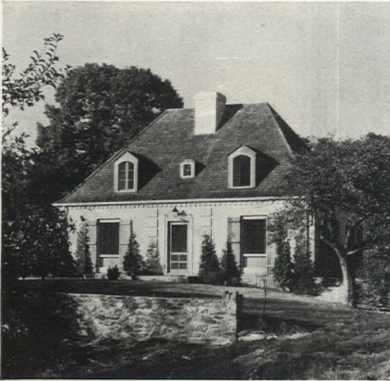
The concrete residence of Earl Katzenstein, Chappaqua, New York. Designed by Emil J. Szendy, New York. Built by O. Berg & Company, Howard Beach, L. I.
