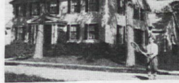
Restored home of Mr. L. W. Longfellow, Machias, Maine. The original house, above, was photographed in 1887
