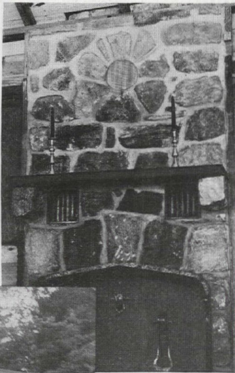
With a cleverly designed system of flues, one chimney serves both the massive inside fireplace and the big outdoor barbecue
