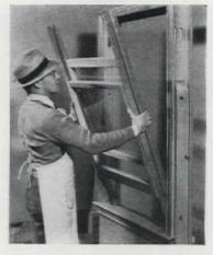
**R**<sup>EADY</sup>-made wood window unit, complete with frame and glazed sash, has weatherstrip and metal sash track built in. Provides insulation and paint free, non-stick contact. N. S. W. Co.
