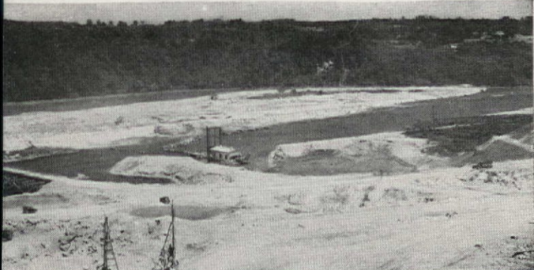
It began with the flood control dam at Franklin Falls
