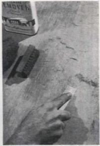
Now on paint remover, let set, remove gummy mass with a putty knife. For carvings use a brush. Clean off wax with naphtha
