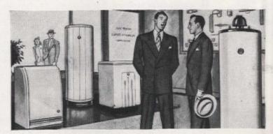
Rheem automatic water heaters, 20 to 100 gallon capacity for any type of gas, including liquid petroleum gas—also models for electricity and oil. All have the patented Rheem-processed tank, which keeps water clean and fresh—guards against rust and leaks. Gas models approved by American Gas Association.
