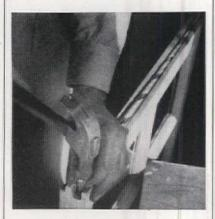
Clide bearing arm to extreme top with screw hole end up. Slip top of balance into drive fastener. Attach lower drive fastener, with flanges down, to bottom of balance and drive
