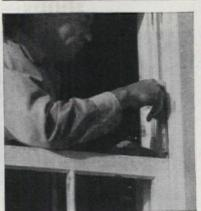
Sash is replaced and bearing arm fastened to jamb. Parting strip and window stops have been replaced. Install 3" stops at top and bottom, make final tension adjustment with wrench or screw driver. Job is done
