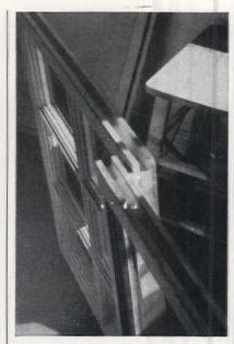
nvizible sash balances were installed in this case; require round bottom groove 5/8" wide by 3/4" deep. Sash are ready for balances. Some makes require a different size groove
