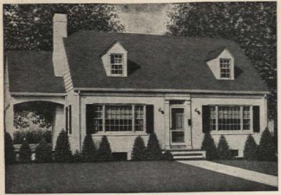
Designed for solid comfort, lasting value. Brick construction, full basement, hot water heat, hardwood floors, complete tile bath. Low cost is made possible by plans standardized to avoid waste.
