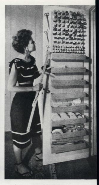
• Example of a closet door at work. The essentials for any sewing job catalogued, available in entire array with one motion of wrist. Bins are made from  $\frac{1}{2}$ 6 inch plywood
