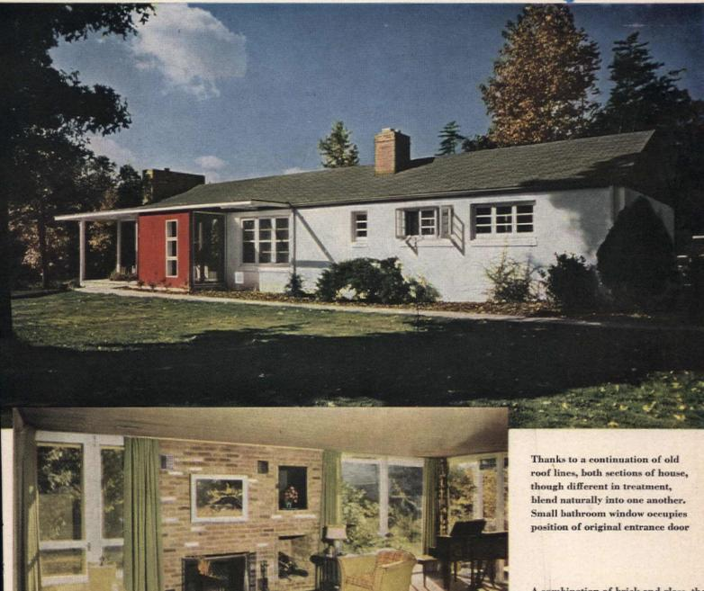
A combination of brick and glass, the new all-purpose room is plenty big— 18 by 26 feet—and tough. Its floor is of flagstone, to accommodate needs of a family with active children. Wall adjoining old house is of birch plywood, ceiling narrow fir boards
