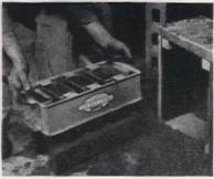
You can mold your own concrete blocks for this shower stall—40 x 44 inches, 76 inches high —and set them in a total of 20 hours. Materials and fixtures came to \$12, plus Kreger Concrete Block Mold (\$12.50), shown in operation
