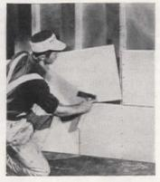
Plaster base of insulation board saves cost of lath for plaster-finished walls
