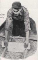
Above, rock wool is blown under attic floor, and mica pellets are spread between open joists. Right, a blanket of glass wool is laid between floor joists
