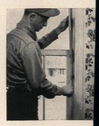
Scrape off excess paint with putty knife, and sand smooth. Plane off extra wood. For free movement and future expansion allowance, a space of 1/16 to 1/8 inch between sash and frame on each side is best. Check sash pulleys or balances for needed repair or lubrication
