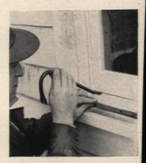
Light and repeated tapping on a wood block along the edge will loosen casement or storm sash with winder or locks open. If the space on the hinge side of a casement is a bit wide, and binding is on the opening side, not top or bottom, set hinges deeper rather than plane sash
