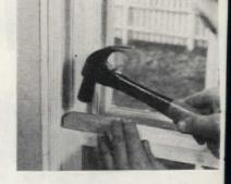
Sticking may be due to warping. Or paint may cause the parting strip to rub against sash check rails. In such a case, tap the strip near where check rails of both sashes meet. This should seat the strip in its proper groove and eliminate the sticking
