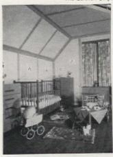
Insulation wallboards do double duty, insulating and finishing wall and ceiling
