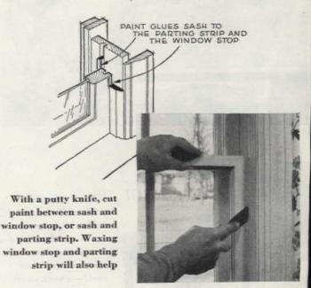
Using a block to protect paint, tap the stile on each side of a double hung sash, firmly but lightly. A gentle shock may loosen any paint that is binding and may move the sash slightly, since windows are seldom closed fully
