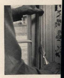
After removing lower sash, a parting strip must be extracted to get upper sash out. Drop upper sash to bottom of frame, and pry out top of parting strip. Then slip strip up and out from behind check rail. Sash cords or balances and weatherstripping must be freed for all sash
