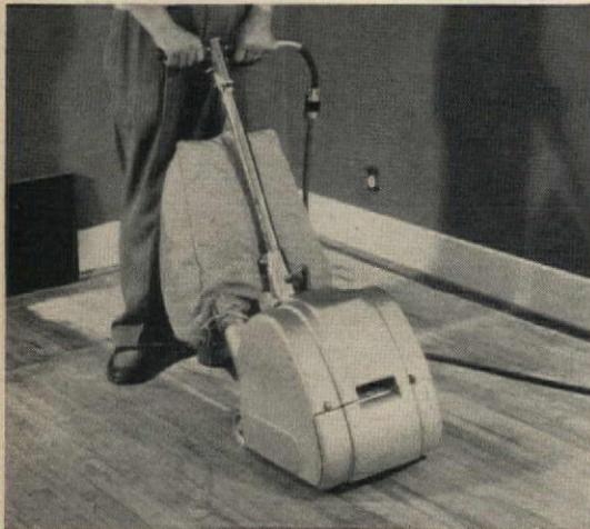
The unsanded floor surface that borders the room is quickly removed with the edger, which operates flush against the baseboard. By moving it briskly in a clockwise pattern, it will smooth off the area to match rest of floor. Use type paper you did on drum sander.
