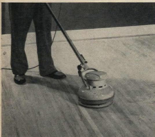
For extra smooth, satin-like finish, disc-sand the floor after drum- and edge-sanding it. This extra sanding makes it much easier to steel-wool floor, and cuts down amount of sealer needed.
