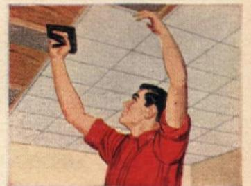
**SOUND-ABSORBING** Gold Bond Insulation Tiles are easy to staple or nail in place. Interlocking edges hide fasteners. Tiles have flame-resistant finish, come in ivory or an assortment of four pastel colors.
