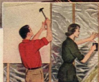
**WALLS GO UP FAST!** Panels of Gold Bond Gypsum Wallboard are easily applied. Saw like lumber, or score with knife and snap! Staple TWINSULATION (rock wool plus aluminum) between studs and rafters.
