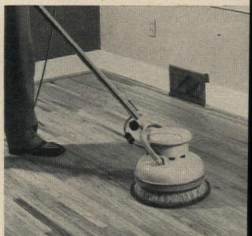
Before first coat of sealer dries completely, a pad of #000 steel wool under brush of rotary sander and go over floor. Then let the floor dry overnight. A second coat of penetrating sealer is recommended for best results on most kinds of wood.
