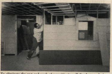
To eliminate the cost and work of repositioning all the ducts and pipes that run through basement, they were hidden by lightweight wood framework that's dropped from ceiling joists and covered with ceiling tile.
