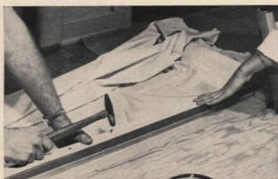
6. Couch is upholstered in 2 layers of fabric, muslin and upholstery. Remove back. Double-fold 2" of muslin, place under front edge of seat frame. Slip cardboard strips between folds to keep fabric from pulling between tacks. Tack along underside of seat frame, from center out to sides.
