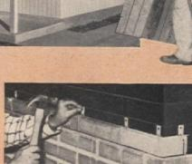
Real-brick veneer is nailed directly to sheathing without clips. Applied to wall, joints of both types of bricks are mortared with trowel or calking gun.
