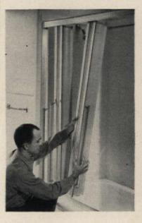
Slip nylon slides at bottom of doors onto rails of tub track, and installation is complete. Door panels come in white, yellow, green, gray, turquoise and peach.
