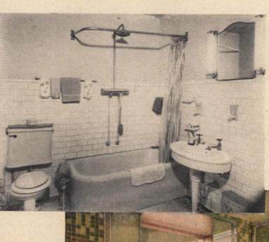
SWITCH-ABOUT BATHROOM in the home of the Charles Martins' is a bathroom remodeling job in which changes in the location of plumbing pipes were kept at a minimum. Fixtures were
