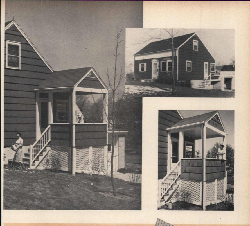
Asbestos-cement shingles in wood-grain pattern are fireproof and durable; can be applied over wood, gypsum or insulation sheathing using metal channels or nails.
