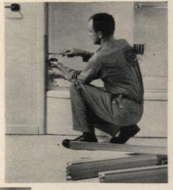
Cut upper track to length, slip nylon sheets of the "Tubmaster" doors into the track and position assembly on jamb posts. Nylon slides, so trolleys operate quietly.
