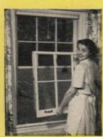
One of the many windows you can consider in remodeling is this double-hung window with sash that tilt in for full, draftless ventilation and that lie flat for easier cleaning. Another double-hung window, above, has removable sash.
