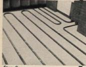
Install radiant panel or grid of steel pipe and connect with existing hot water heating system.
