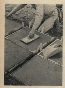
smooth concrete with wood float, then an hour later, with steel trowel. Stroke trowel from edges to center to make a slight crown to shed rain. Use packaged, dry-mix concrete or mix concrete in a wheelbarrow using one part cement to two parts sand to three parts of gravel.
