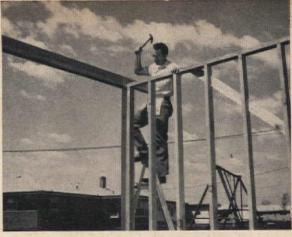
ONE OF THE FIRST STEPS in building the garden house is the erection of the 2x4" frame walls. Horizontal plate is nailed to vertical studs. Bottom ends of the studs are nailed to sill which in turn is bolted to the concrete slab. A large beam spans screen opening.
