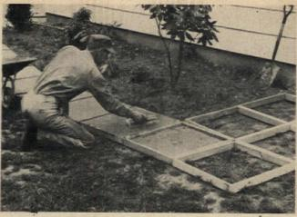
cast-in-place-slabs follow contour of ground underneath so they won't jiggle or rock. Before pouring concrete, remove high or low spots; tamp earth with back of shovel.
