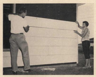
ONE OF THE LAST STEPS in finishing the garden house is application of the primed hardboard, clapboard siding. An aluminum mounting strip nailed to the framing holds each course of siding in place. There are no exposed nail holes. Siding received two coats of paint.
