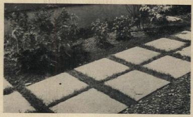
FINISHED WALK is very practical and permanent. The forms can be lifted from concrete slabs about 48 hours after placement. Spray the slabs and sod for four days for strong concrete and healthy grass.
