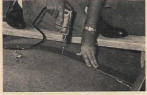
5"-wide strips of 3/16"-thick tempered hardboard. Strips are fastened to end of panels with nuts and bolts. Roof is then coated with aluminum paint.
