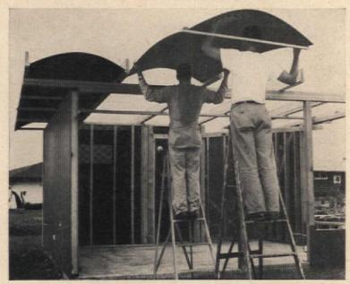
ROOF PANELS of 3/16"-thick tempered hardboard are inserted between the beams and slid along in the slots on the wood strips that are nailed to the beams. The special flexing frame keeps the hardboard panel in line so that it's easy to handle and insert into the slotted strips. Metal strapping along bottom edge of the beams keeps them aligned. A 1x12" board fascia is nailed to the outside edge of the roof and all joints are filled with water-resistant calking compound.
