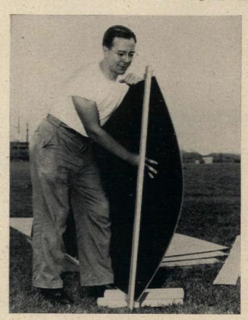
TEMPERED HARDBOARD PANELS that make up the sections of the roof are four feet wide and ten feet long. Tempering makes the panels impervious to rain. To prepare the panels for insertion between the roof beams they are flexed and held in a special frame made out of a board with a block of wood at each end. This frame curves panel to fit between beams.
