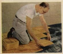
Easy to lay—Bruce Blocks may be installed with an adhesive over any smooth surface or nailed to a wood subfloor or old floor.
