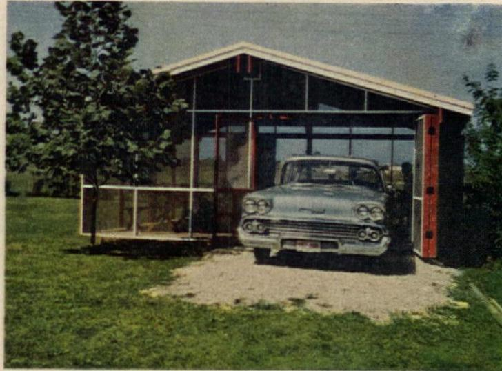
**THE CARPORT DOOR** is made in 3 parts with one section doubling as the entry door. All three fold back to give you a full-sized opening to admit your car. An overhead-acting screen door can also be used. Fiber-glass screening for the house is permanently fastened to the 2 x 4 framing.
