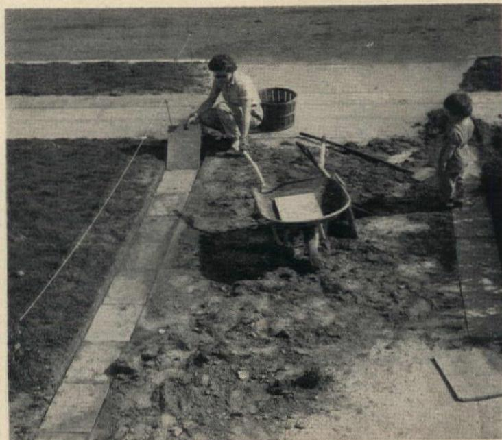
**THE DRIVEWAY**, we decided, was too narrow. So we widened it on each side with rectangular flagstones. We set the stones on several inches of well-tamped gravel plus a layer of sand.
