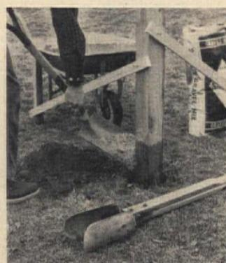
**BEST WAY** to place a vertical post is to set it in its hole, then brace it in two directions. Use a spirit level on one face of the post, then anchor and nail the brace. Move 90 degrees, use the level again, and nail the other brace. For a permanent installation, fill the hole around the post with tamped gravel-mix concrete.
