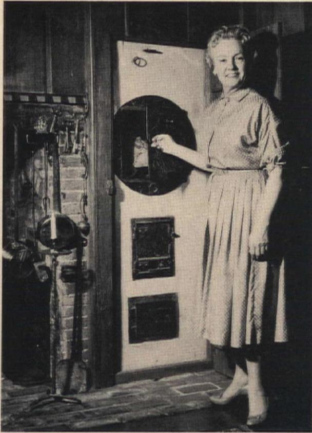
**BUILT-IN WALL OVENS** aren't really new, as Mrs. Chamberlain points out here. This is a Count Rumford oven and was probably installed in the late 18th Century. Original bake oven inside fireplace was holed up. Note the firebox and receptacle for ashes underneath the oven.
