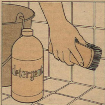
Scrubbing stains off tile (page 16)
