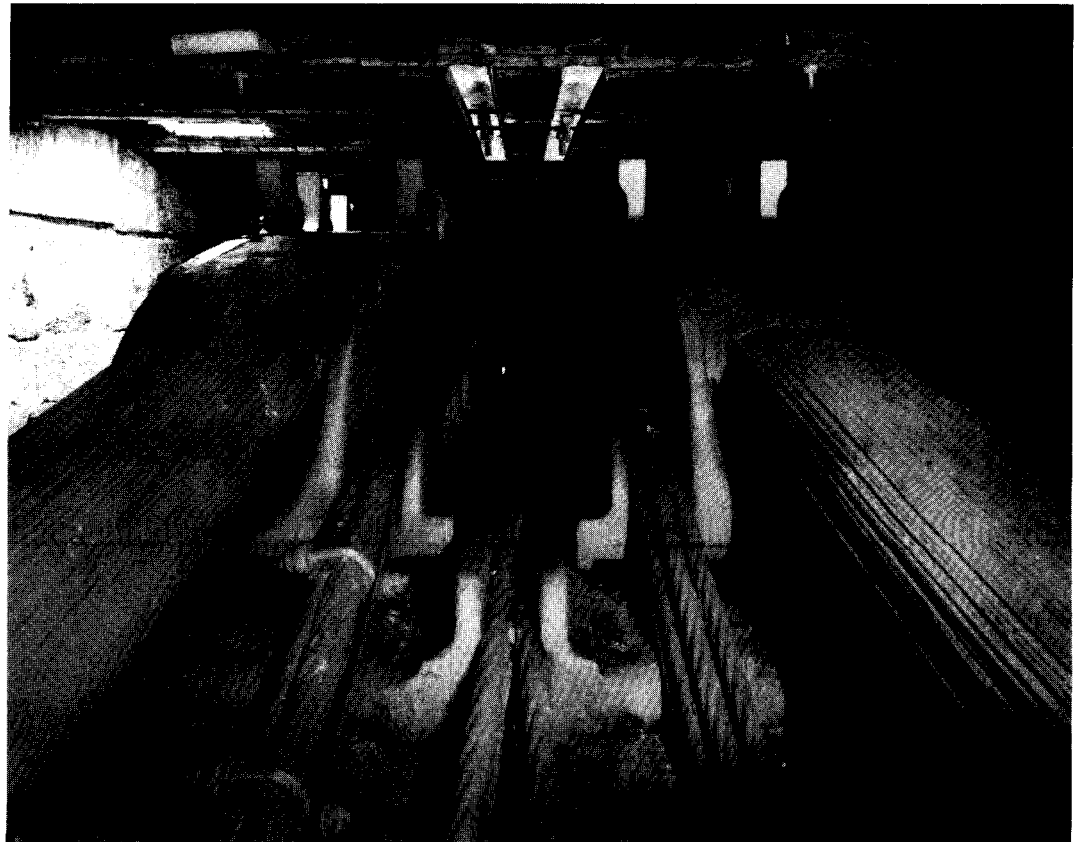
Above, aerial view of the top of the bridge's Brooklyn tower. Right, center saddle of the Brooklyn tower bearing cables. Across page, detail of diagonal stays beneath roadway.
