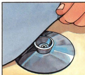
1 Roll membrane over knobbed base plate.
