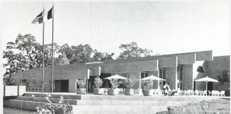
Piper Sonoma Cellars , Healdsburg, California Jury Comments: "It's very refreshing to see a winery treated like this. This is a very nice use of concrete and the glass gives it a lighter look. Elegant." Owner: Piper-Sonoma Cellars, Inc., Healdsburg, California Architect: Roland/Miller/Associates, Santa Rosa, California Structural Engineer: Zucco Associates, Santa Rosa, California General Contractor: Paul V. Wright, Inc., Santa Rosa, California
