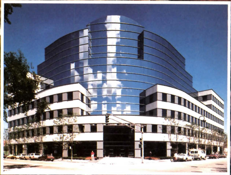
Stone curtainwall system application by Flour City to the dramatic Shand Morahan Building in Evanston, Illinois. Architect: Murphy-Jahn, Chicago, Illinois.
