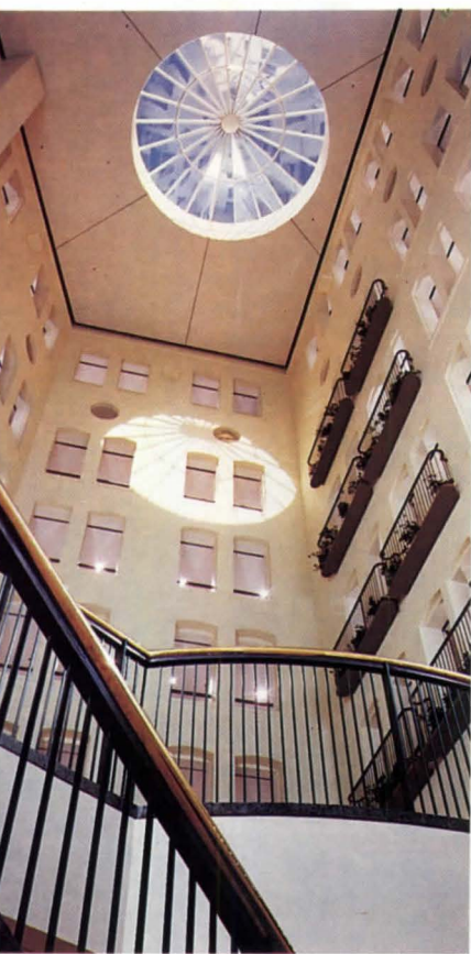
Left, the renovated facades at the intersection of Broadway and Houston. Cor- between the fourth and fifth and fifth six stories are terra-cotta; the top one essed metal painted to match. Near renovated storefronts and a 'before' . Above, round holes under top floor late atrium. Right, glass pavers in e leading from entrance to elevators t from below.
