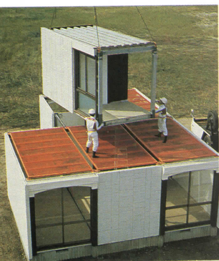
bove, workers set volume—complete with doors, windows, interior finishes, and services—into place. All of the volumes of a house can be positioned in less than an hour. Two more weeks of construction are required (for wiring, plumbing, and finishing work) before a house is ready for occupancy, right.
