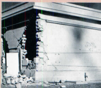
Shear forces generated by seismic ground motion, wind, and snow load are especially devastating to rigid structures. Because wood-frame design is more elastic, it dampens these stresses, leading to improved seismic stability.
