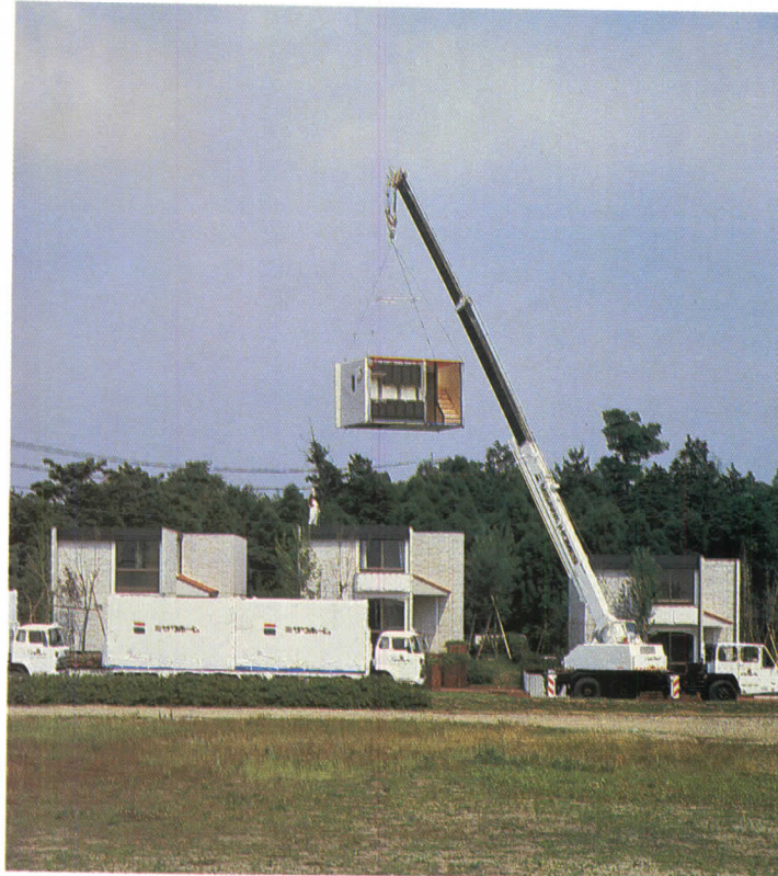
Above, conventional poured-in-place concrete footings support prefabricated volumes, which are transported to the site on trucks. Right, local subcontractors, affiliated with Misawa, hoist volumes from truck using a separate crane. Most houses are comprised of seven to ten volumes. The size of each volume is limited by road transportation restrictions.
