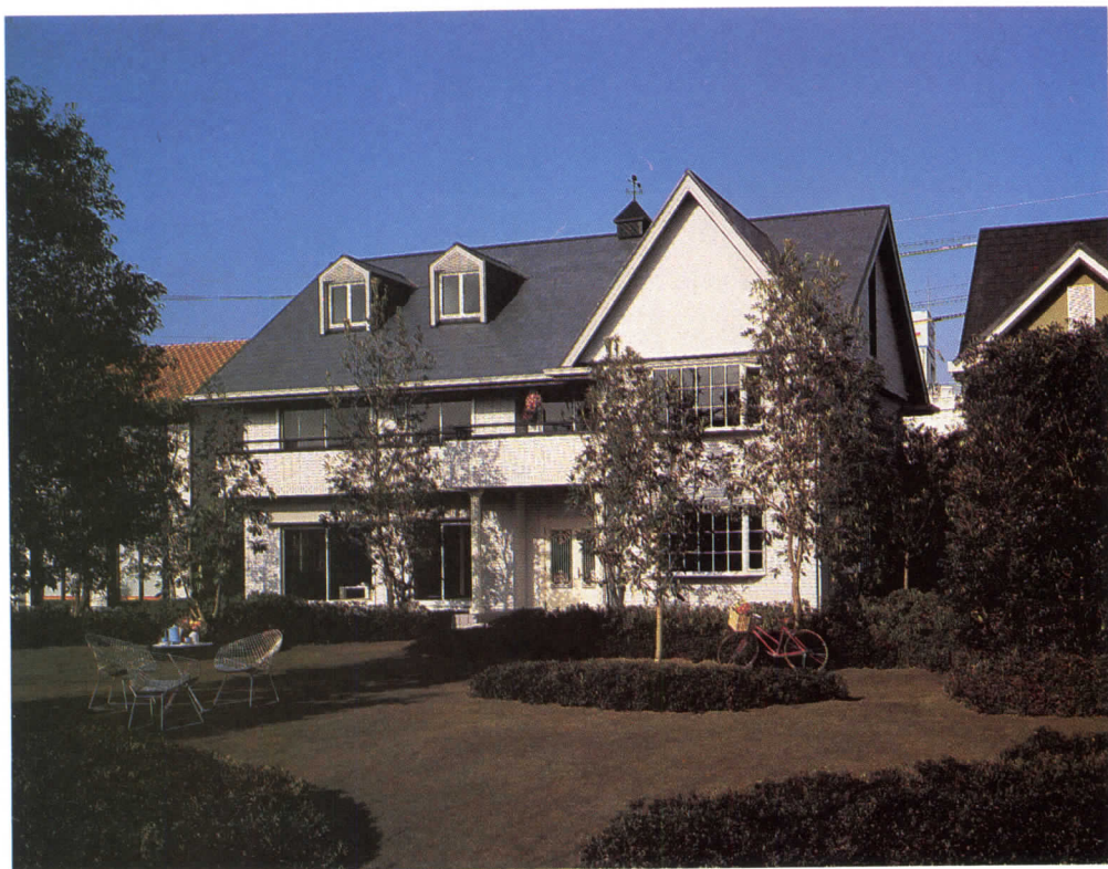
bove, workers set volume—complete with doors, windows, interior finishes, and services—into place. All of the volumes of a house can be positioned in less than an hour. Two more weeks of construction are required (for wiring, plumbing, and finishing work) before a house is ready for occupancy, right.
