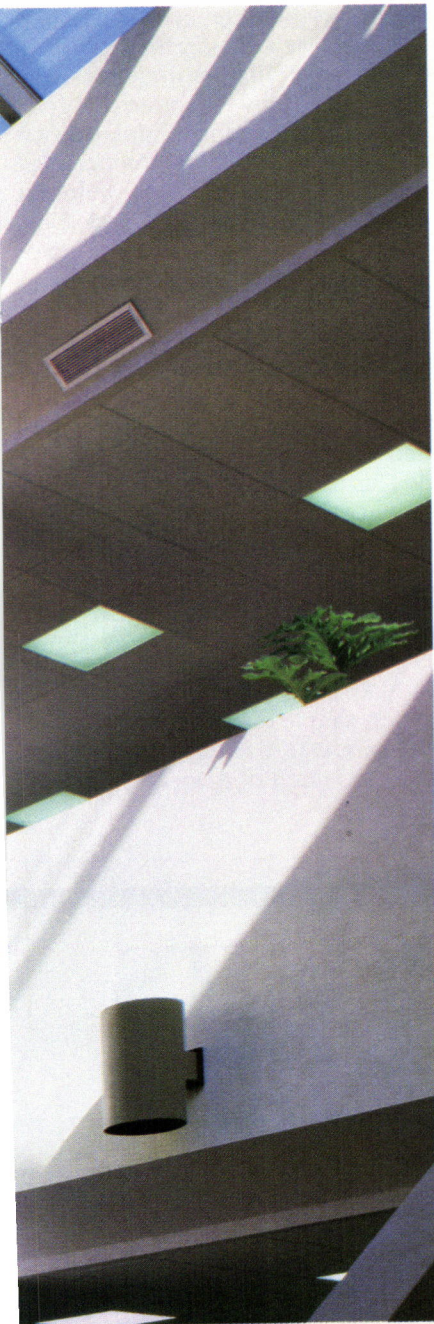
STANDARD GRID with its wide 1 5/16" exposed face provides for a ceiling design that is coarse by today's standards. Shown above with standard square-edge lay-in panels.
