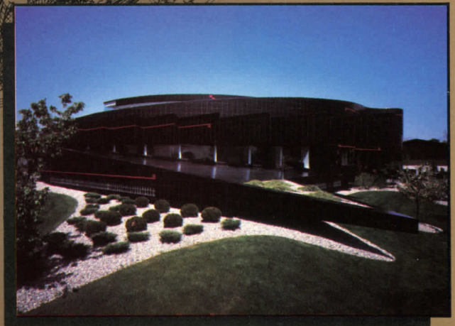
Architect: Harvey Ferrero Roofing Contractor: Brodak Roofing & Sheet Metal Carlisle Manufacturer's Representative: Holmes Associates
