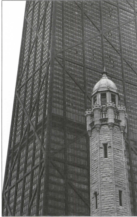
Figure 1, left, graphs the weights per square foot of steel needed for floors, columns, and wind versus number of floors in a building. Chicago's Hancock tower, above, was designed to keep these steel requirements to a reasonable level. Figure 2, below, compares actual stress due to shear lag versus true cantilever stress.
