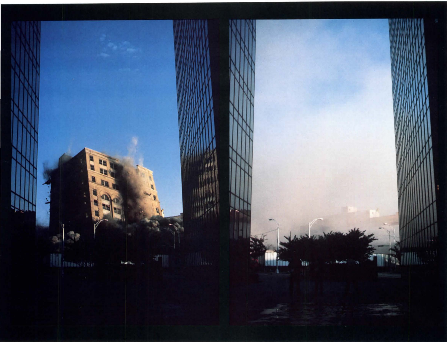
Photographs courtesy of Controlled Demolition Inc.
