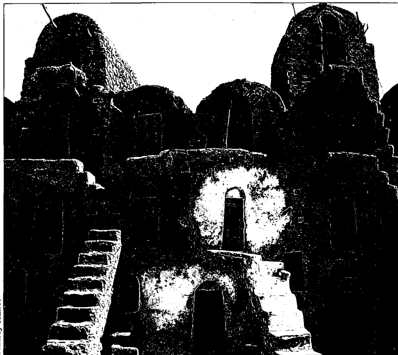
Stairways and four-story grain storage vaults in Tunisia.
