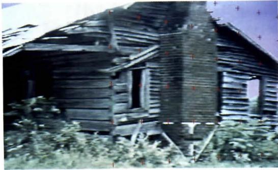
Video images are measured via overlaid stadia, right; then are converted to CADD, right below.
