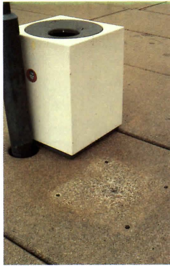
Photos indicate the minor repairs needed as the Opera House marks its 16th birthday. Note the state of the tiles in the two photos to the far left. The photos directly above and to the immediate left show concrete damage; discarded cola in trash can ate the concrete finish below it. Far right photo shows ponding at stair.
