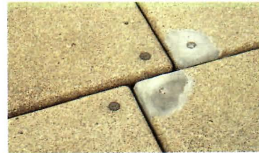
Photos indicate the minor repairs needed as the Opera House marks its 16th birthday. Note the state of the tiles in the two photos to the far left. The photos directly above and to the immediate left show concrete damage; discarded cola in trash can ate the concrete finish below it. Far right photo shows ponding at stair.
