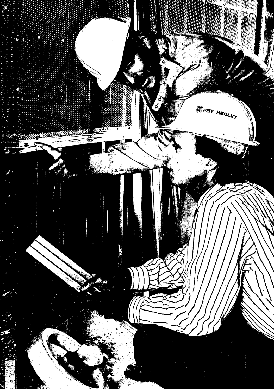
Fry representative consults on site of Library Tower project, Los Angeles, California. I.M. Pei & Partners, Design Architect. Ellerbe Becket, Executive Architect.
