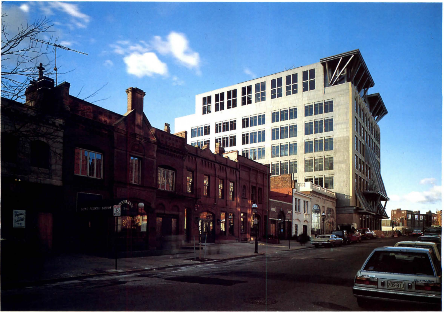
Above, the jagged silhouette from the approach down Newbury Street. Right, the building over the Massachusetts Turnpike.
