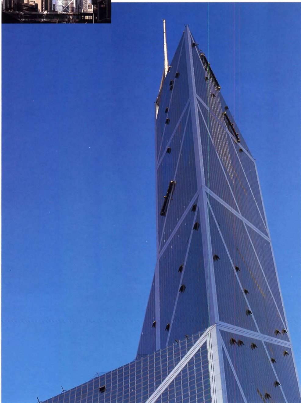
Reflective glass saves energy while aluminum cladding expresses structure.
