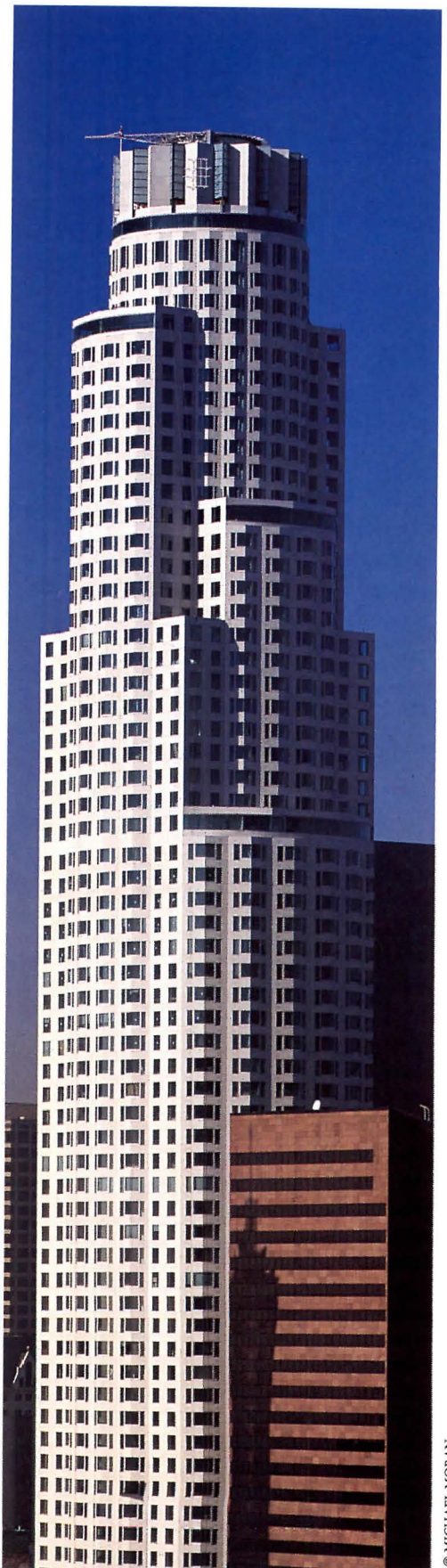
Setbacks at the 48th, 61st, 69th, and 73rd floors give the First Interstate World Tower its distinctive profile, and complicated its structural analysis.
