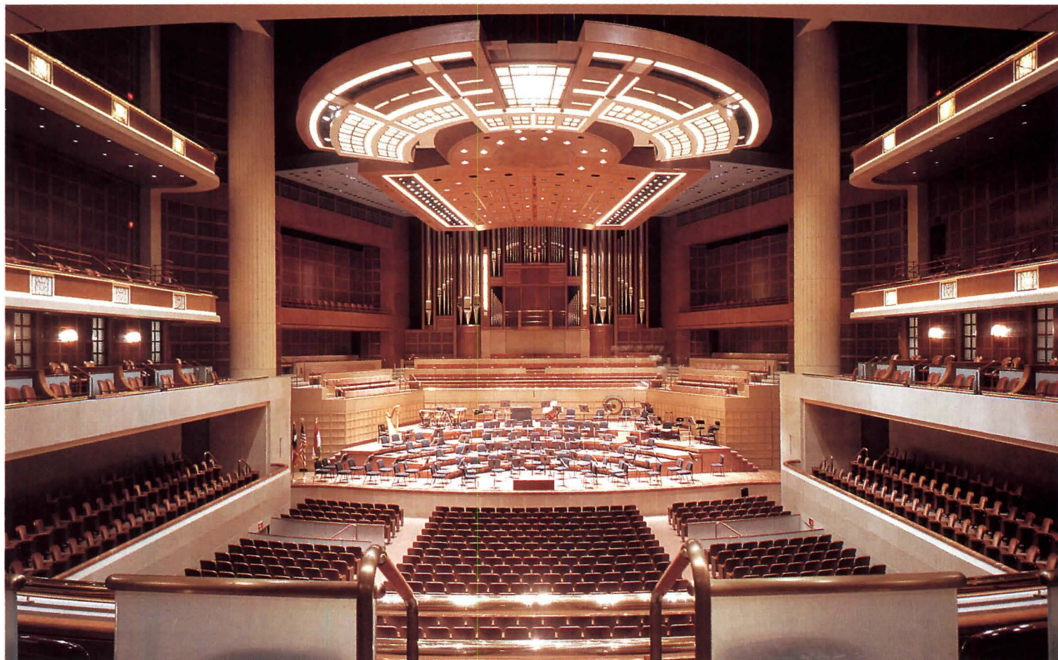
The hall's sound-reflecting canopy adjusts from 40 to 75 feet above the stage and tilts approximately 7 degrees.
