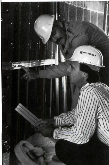
Fry representative consults on site of First Interstate World Center project, Los Angeles. I.M. Pei & Partners, Design Architect. Ellerbe Becket, Executive Architect.
