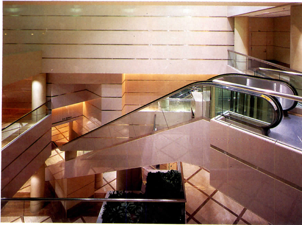
Neopariés panels inside the Delta Air Lines terminal (above) are supported by exposed, stainless steel bands and pinned by stainless steel dowels (detail below). Clip angles behind the panels are bolted to channels welded to the building's steel framing to meet seismic codes.
