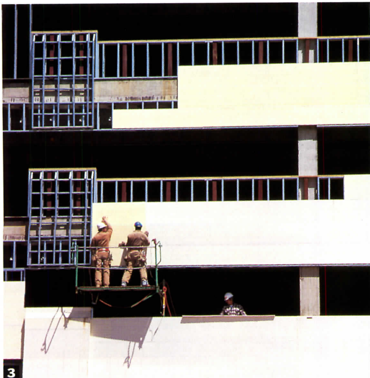
1. Harditexture exterior sheathing looks like stucco and can be used in molding and trims. James Hardie Building Products. Circle 411 on information card. 2. Multi-use, non-asbestos, fiber cement interior and exterior building panels are available from FibreCem Corporation. Circle 412 on information card. 3. Dens-Glass Gold sheathing combines a fiberglass mat surface with a silicone-treated gypsum core and an alkali-resistant surface coating to resist weathering. Georgia-Pacific. Circle 413 on information card.
