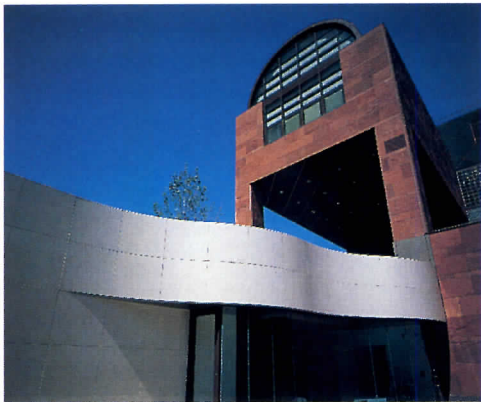
Japanese architect Arata Isozaki specified Neopariés to clad the undulate fascia near the entrance to the Museum of Contemporary Art in Los Angeles (above). Neopariés, compared with marble and granite (below), offers differences and similarities in properties.
