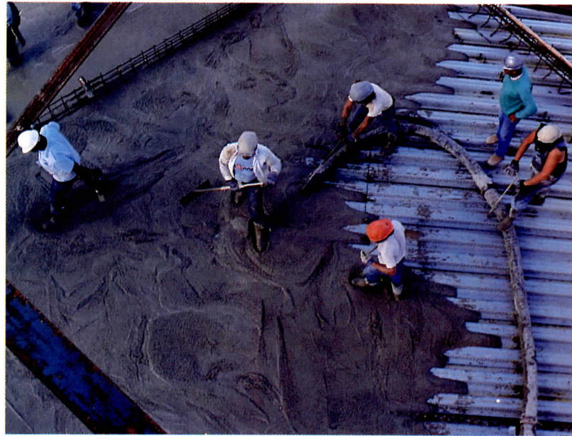
Installing Vulcraft composite deck is faster and more economical than poured-in-place concrete.
