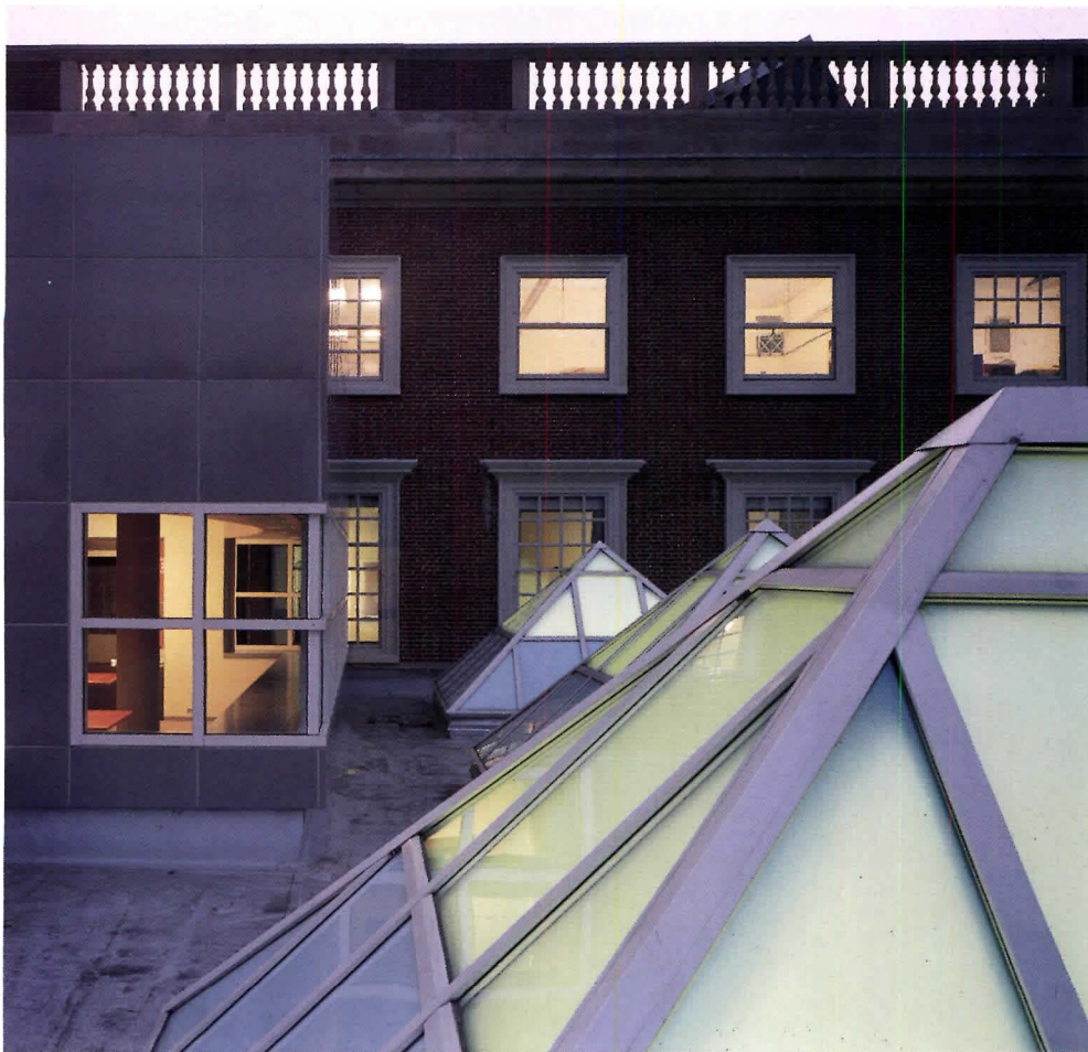
Third-floor study area in south wing (bottom left and plans, facing page) overlooks roofscape of skylights (left) that tops Busch-Reisinger galleries. Fine Arts Library reading room (facing page) is furnished with Gwathmey Siegel-designed tables.
